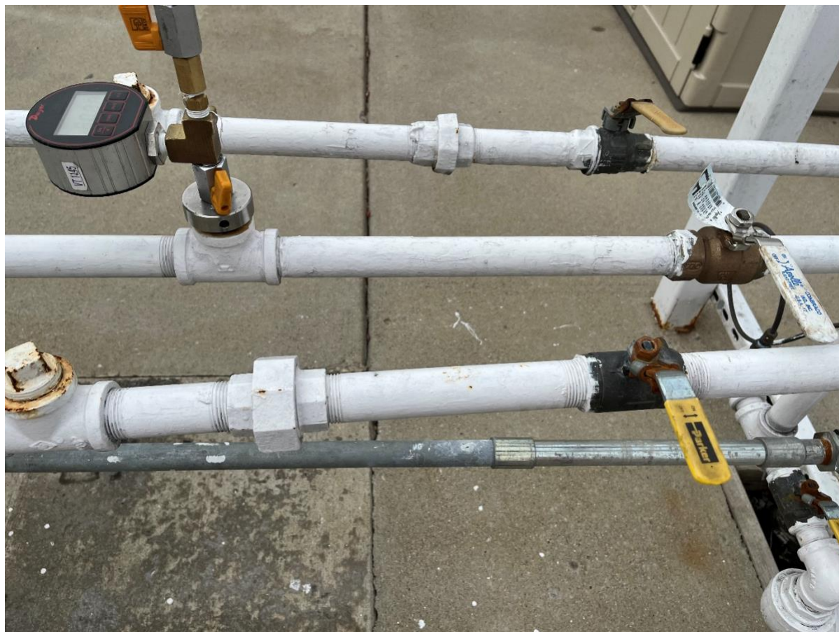
Figure 9-28: GREEN MACHINE leak test
