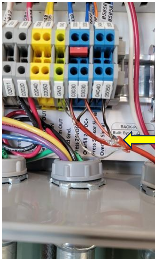
Figure 3-5: GREEN MACHINE Control Panel Connections
