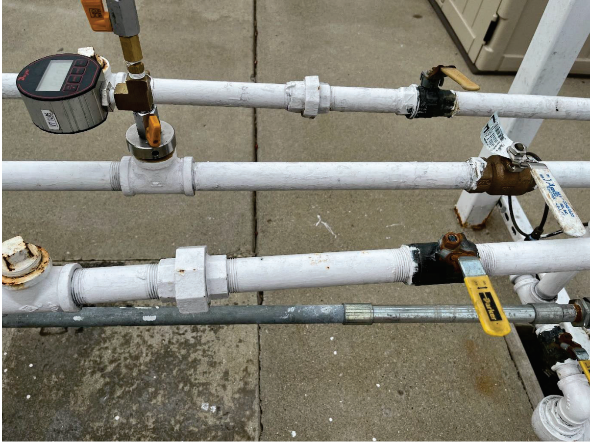
Figure 9-28: GREEN MACHINE leak test
