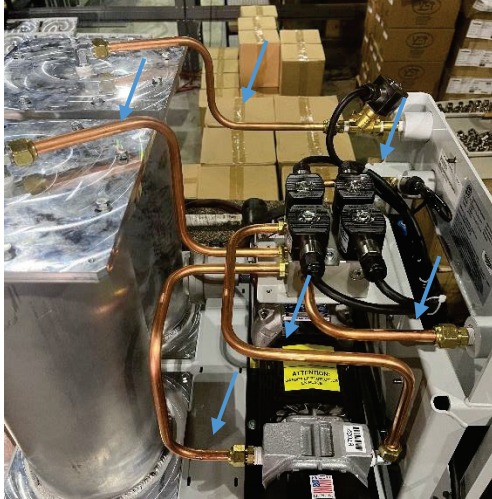
Figure 9-11: Piping to be removed
