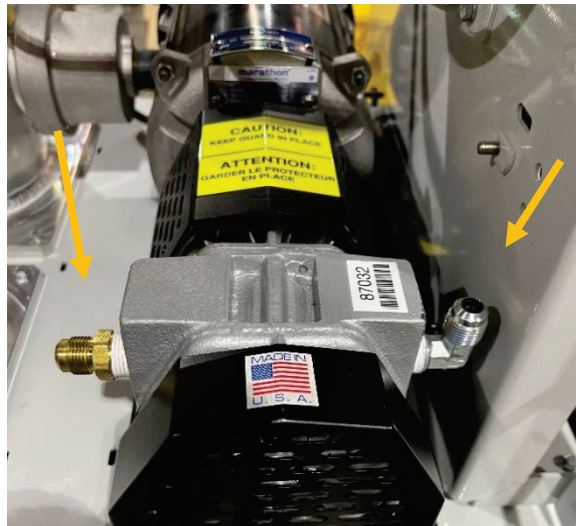
Figure 9-6: Two tubes removed from vacuum pump
