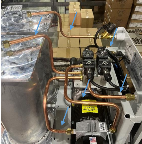
Figure 9-11: Piping to be removed
