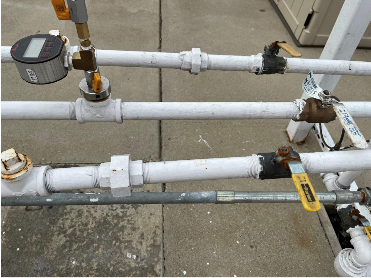
Figure 9-28: GREEN MACHINE leak test
