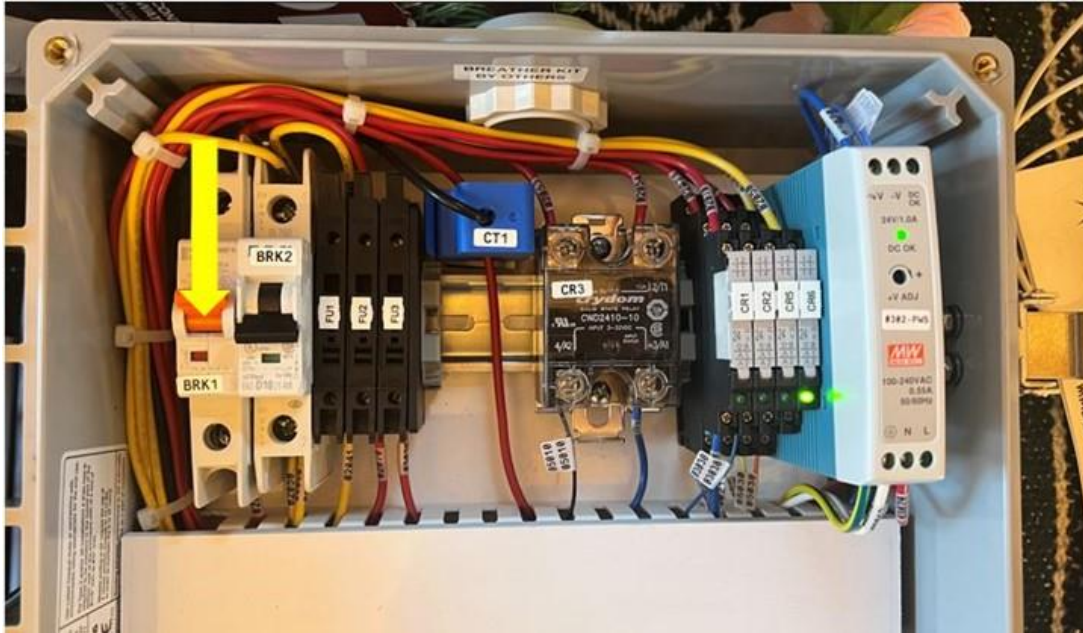
Figure 9-3: Bomba de vacío BRK1
