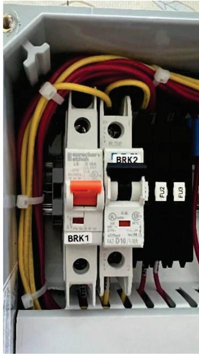
Figure 8-19: Dispenser Bypass Shutdown Breaker (BRK2) is Up (CLOSED)
