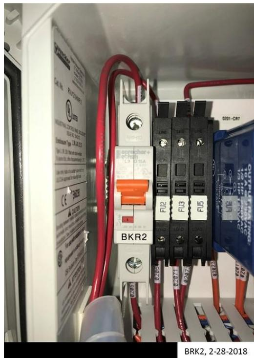
Figure 9-8: Vacuum Pump BRK2
