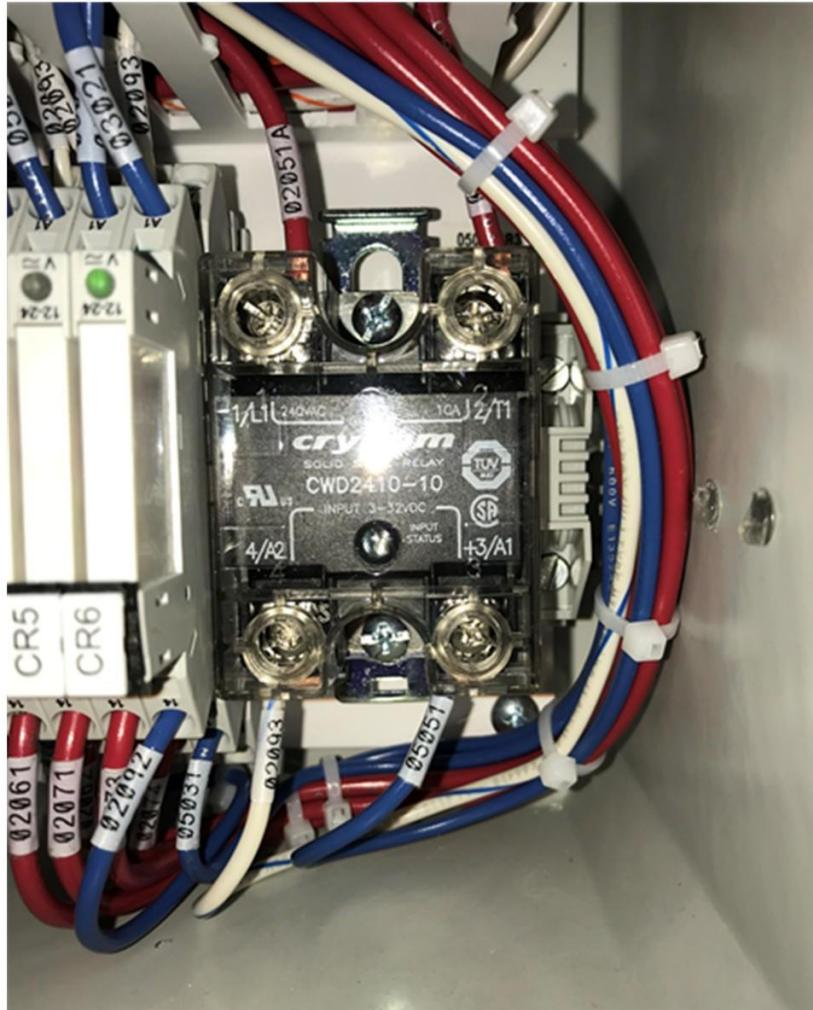
Figure 9-9: Vacuum Pump Solid State Relay
