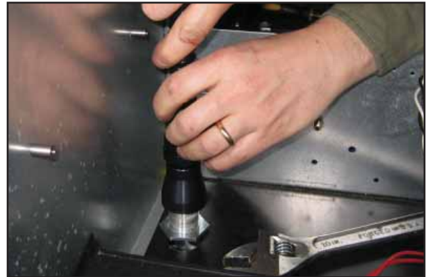
Figure 13: Attach Flexible Conduit
