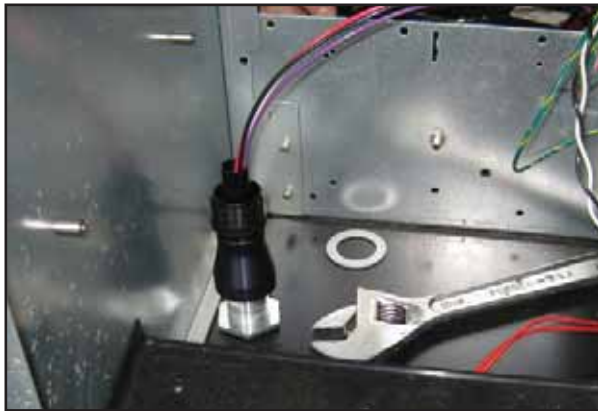
Figure 6: Straight Conduit Installed
