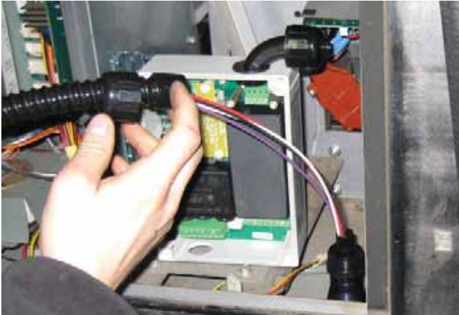
Figure 10: Attach Flexible Conduit to Potted Nipple
