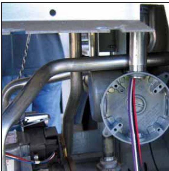
Figure 8: Junction Box Connected to Potted Nipple
