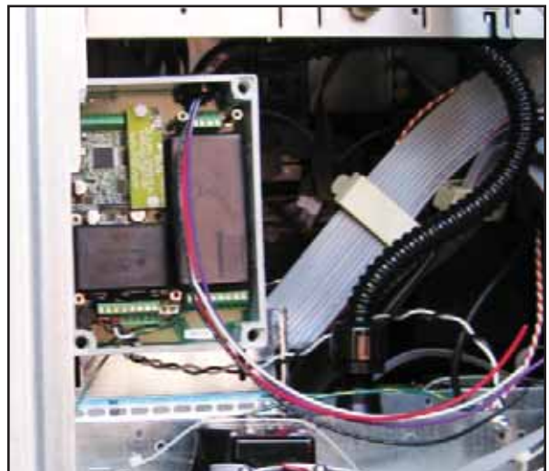
Figure 13: Wires in Flexible Conduit
