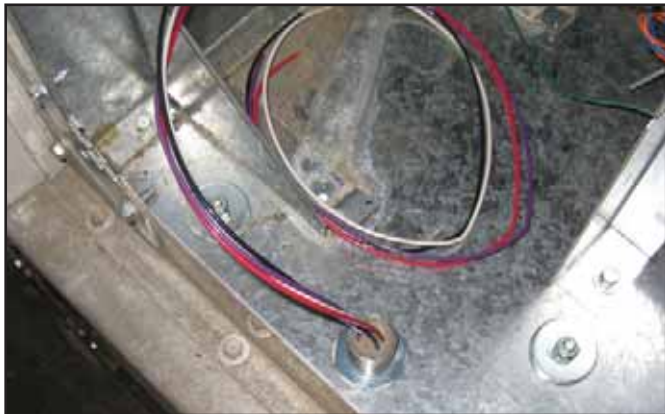
Figure 11: Install Potted Nipple
