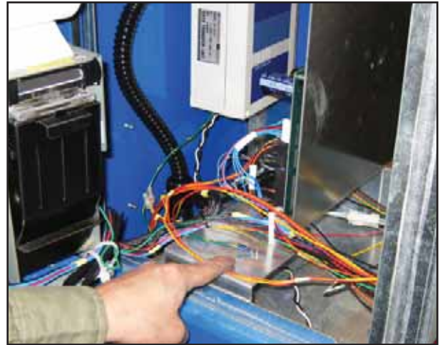
Figure 18: Ground Wire Attached
