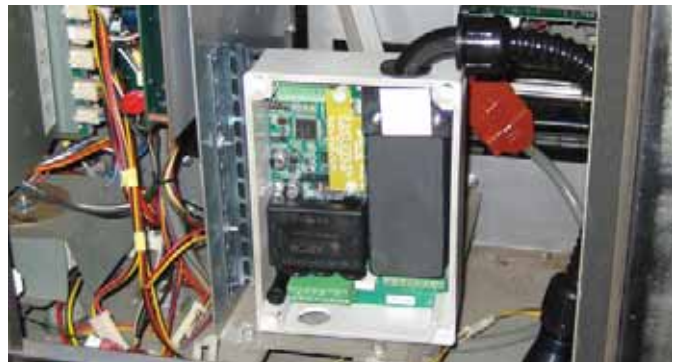
Figure 13: Reinstall Barrier Cover
