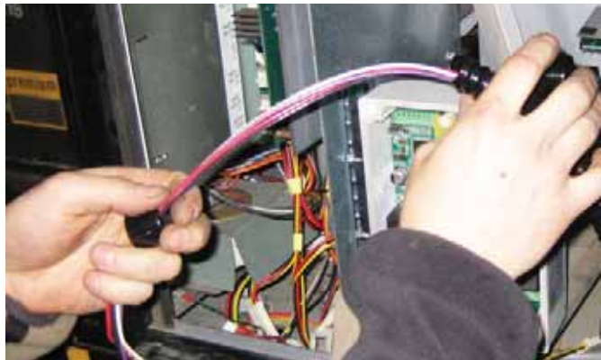
Figure 11: Attach Flexible Conduit to 90-Degree Fitting
