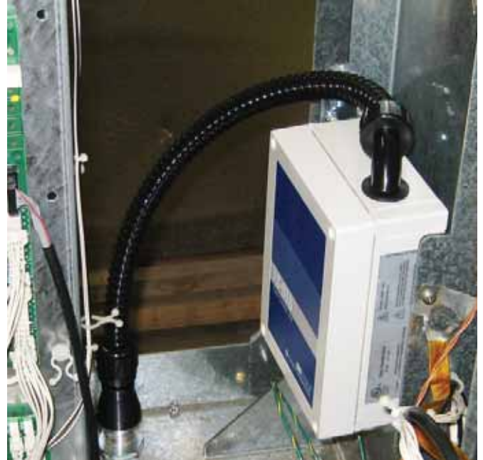
Figure 17: Attach Cover to DTU
