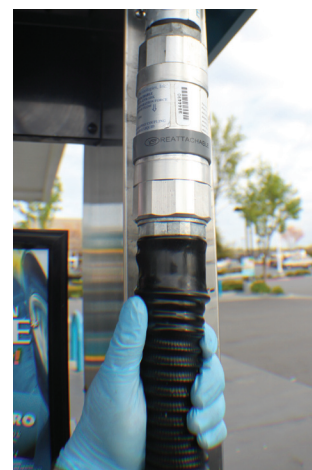
Figure 9: Verify Connection Integrity
