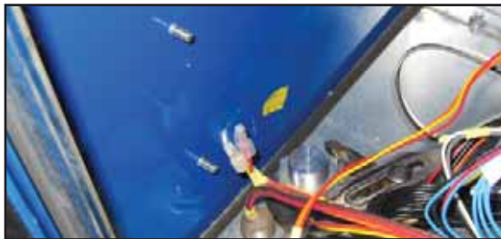
Figure 6: Remove Nut
