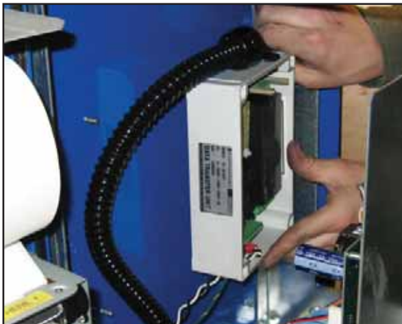
Figure 13: 90-Degree Conduit Connected
