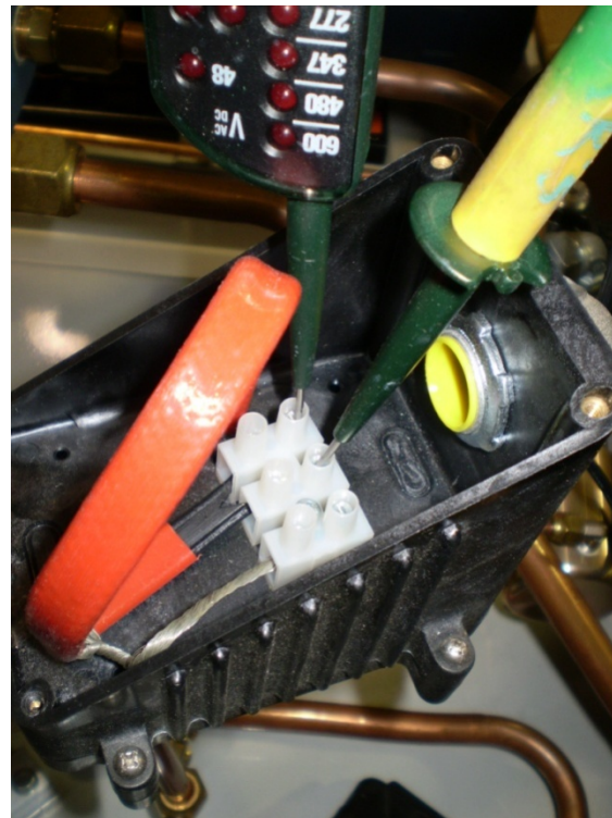
Figure 16: Heat Trace Circuit Test
