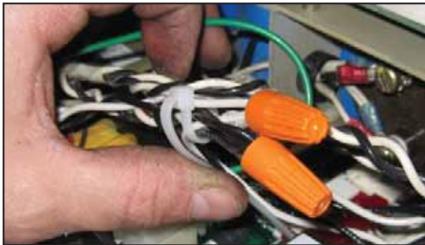
Figure 12: Wrap Wires
