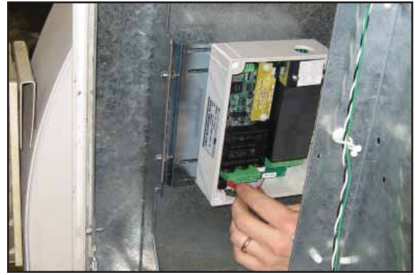
Figure 3: Attach DTU to Dispenser
