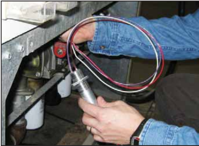
Figure 10: Push Wire to Electrical Enclosure
