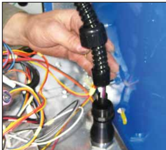
Figure 10: Wire in Flexible Conduit
