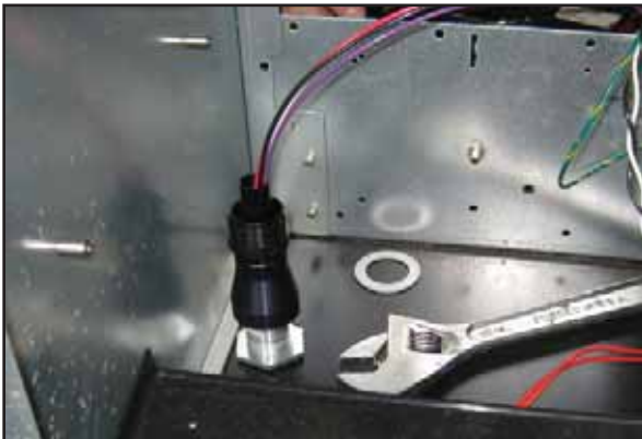
Figure 6: Straight Conduit Installed
