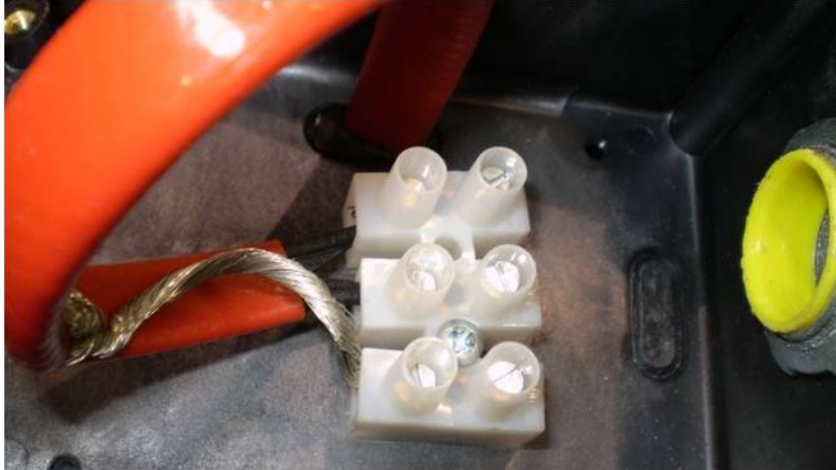
Figure 37: Termination block inside the electrical junction box
