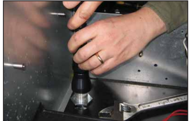
Figure 14: Attach Flexible Conduit
