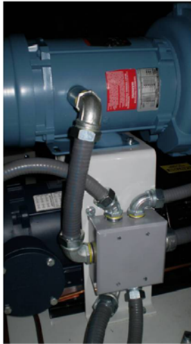
Figure 23: Blower electrical connection conduit
