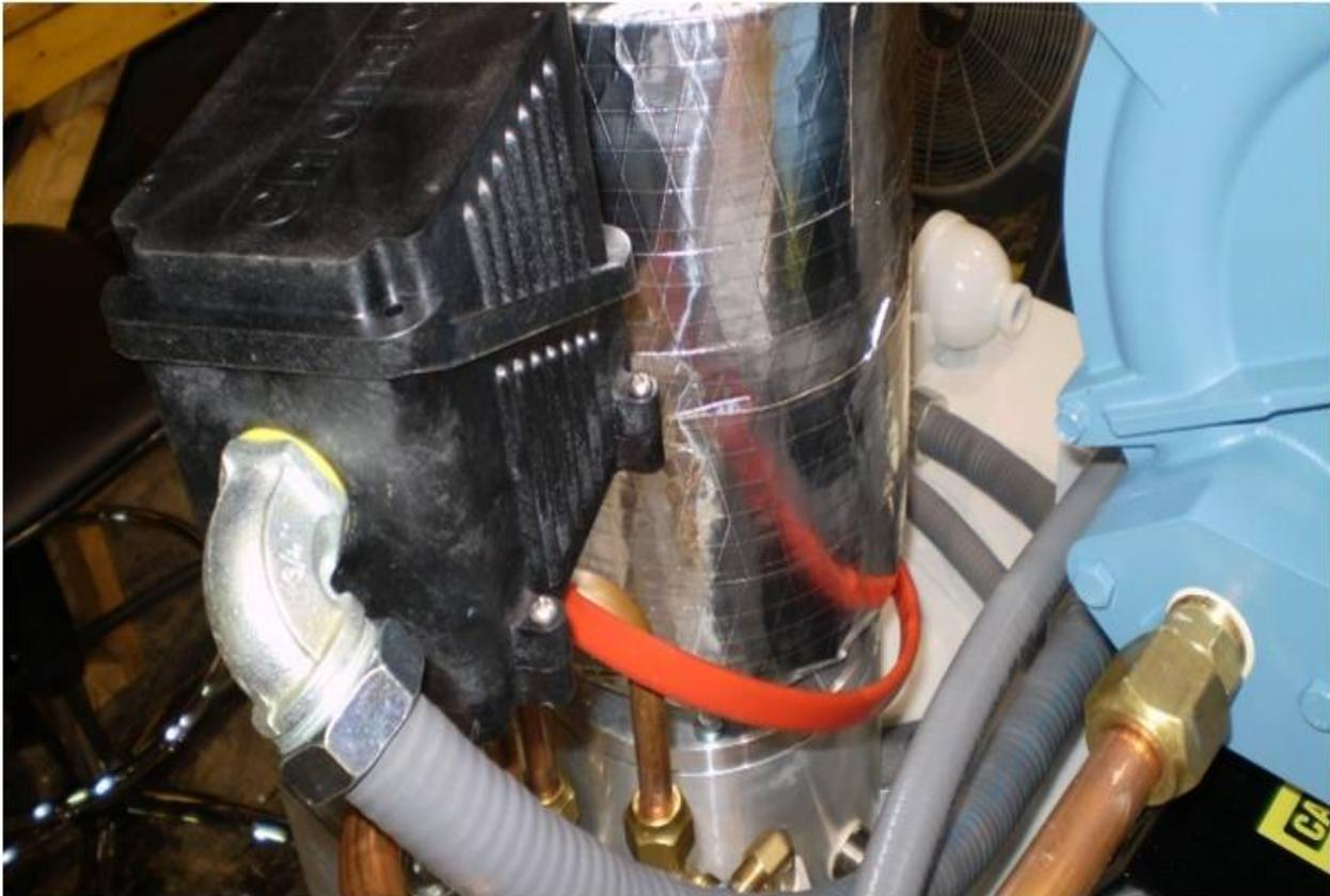
*Figure 48: Installed electrical junction box with electrical connections*
