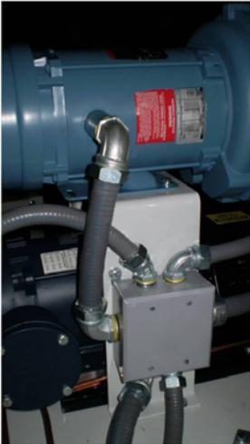
Figure 23: Blower electrical connection conduit
