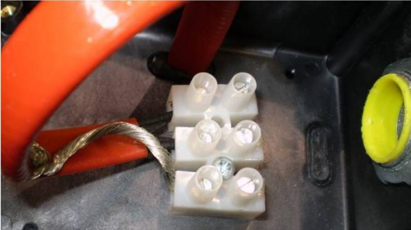
Figure 37: Termination block inside the electrical junction box
