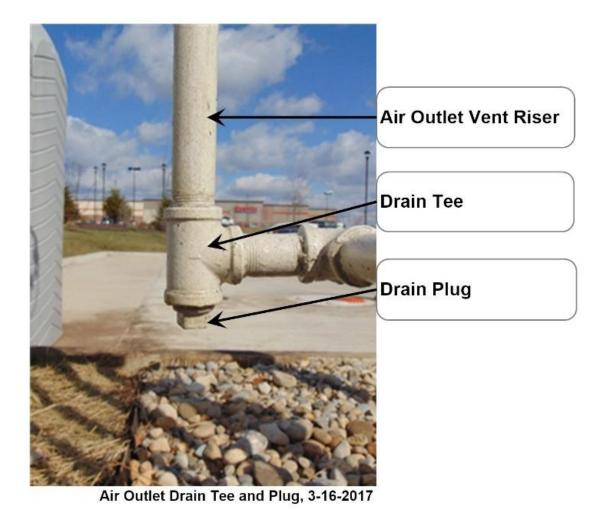
Figure 7-17: Air Outlet, Drain Tee, and Plug
