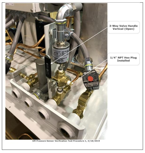
Figure 7-8: Pressure Sensor & 3-Way Valve, NORMAL Operation
