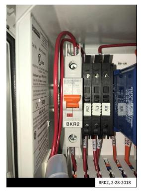
Figure 9-8: Vacuum Pump BRK2
