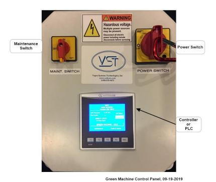
Figure 3-3: VST CS2 Control Panel w/Carabiner Clip Installed
