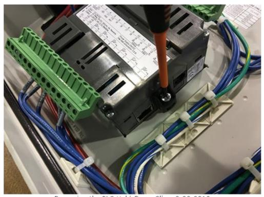
Removing the PLC Hold-Down Clips, 2-28-2018
