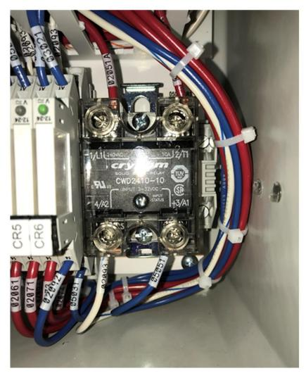
Figure 9-9: Vacuum Pump Solid State Relay
