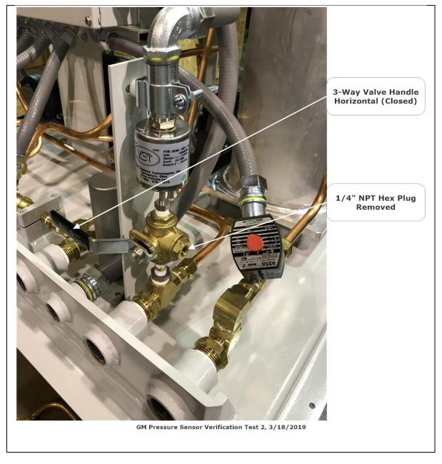
Figure 7-9: Pressure Sensor & 3-Way Valve, TEST Position
