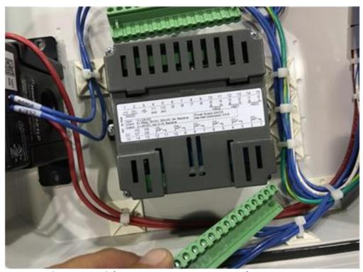
The PLC with Connectors Removed, 2-28-2018
