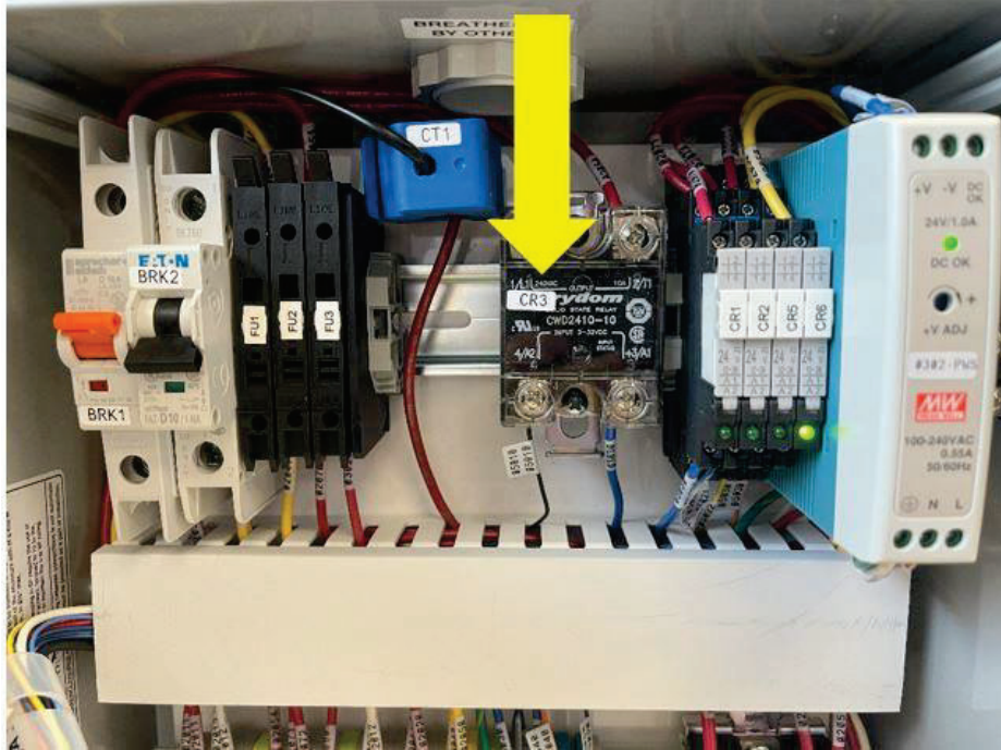
Figure 9-4: Vacuum Pump Solid State Relay
