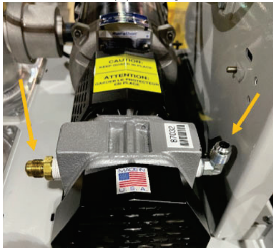
Figure 9-15: Two Tubes Removed from Vacuum Pump
