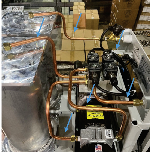
Figure 9-12: Piping to be removed
