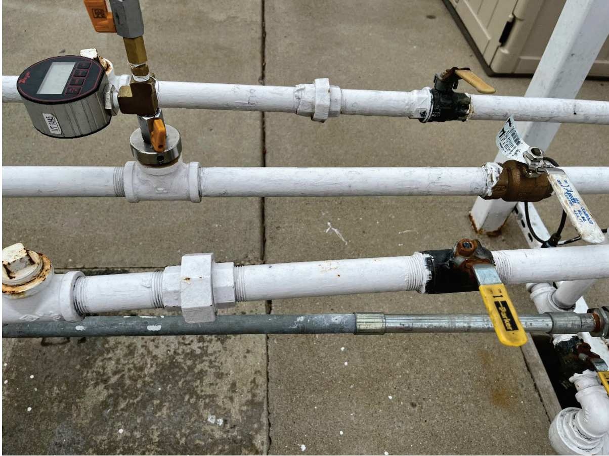
Figure 9-29: GREEN MACHINE leak test
