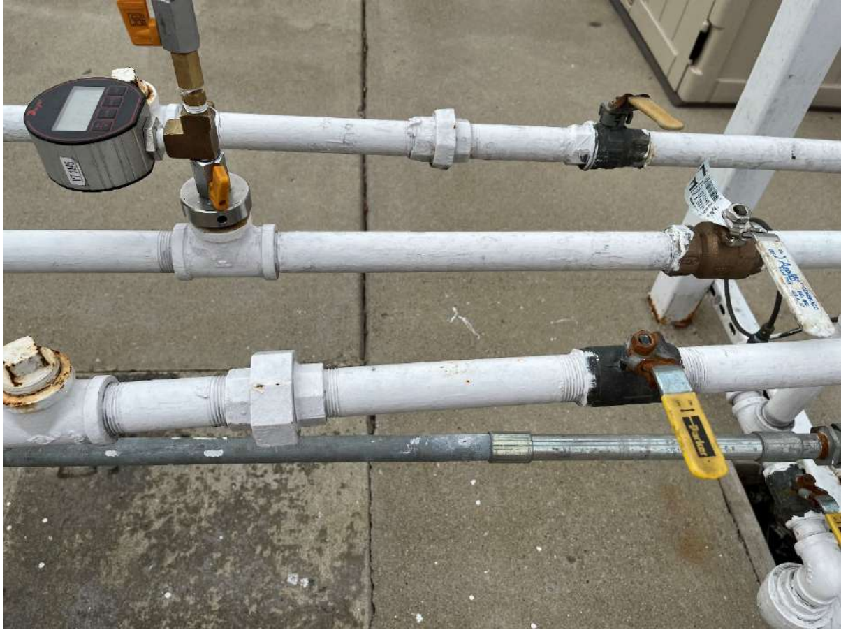
Figure 9-29: GREEN MACHINE leak test
