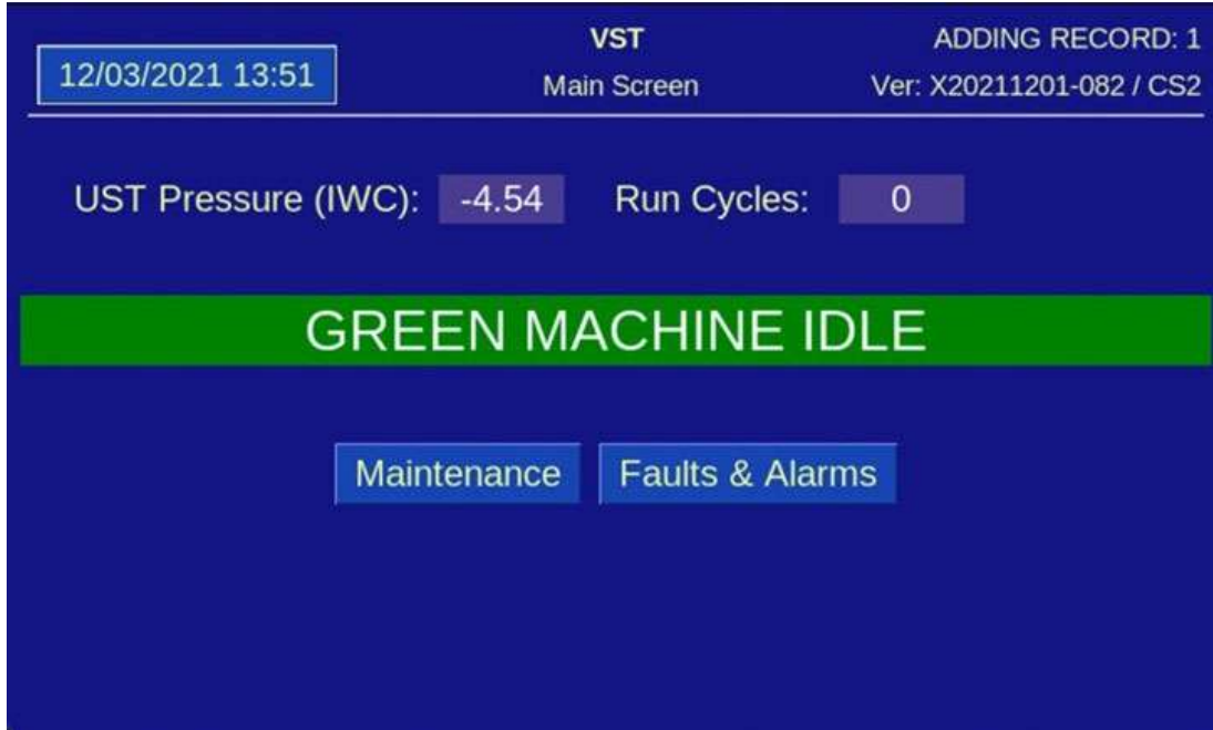
Figure 7-1: VST PLC Main Screen w/no Alarms
