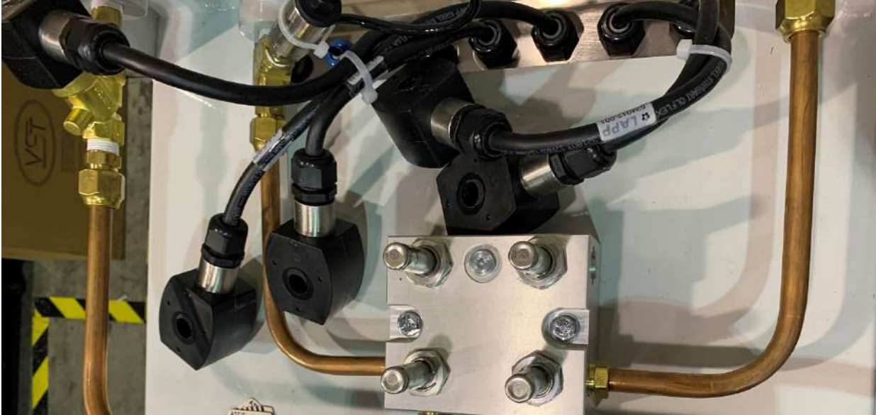
Figure 9-20: Manifold with the Solenoids Removed, showing the Solenoid Bases
