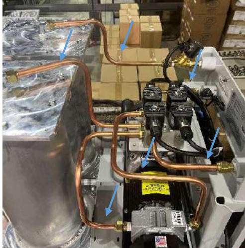
Figure 9-12: Piping to be removed
