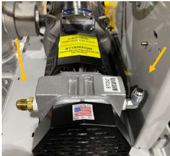
Figure 9-7: Two tubes removed from vacuum pump
