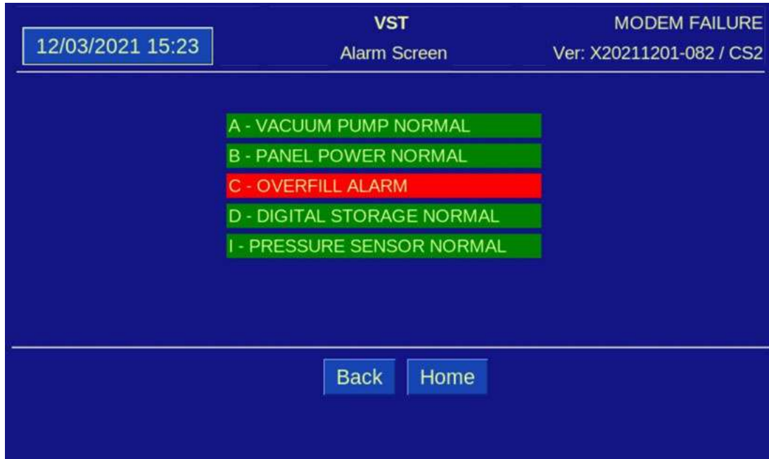
Figure 8-3: VST Control Panel Alarms and Faults Screen Example
