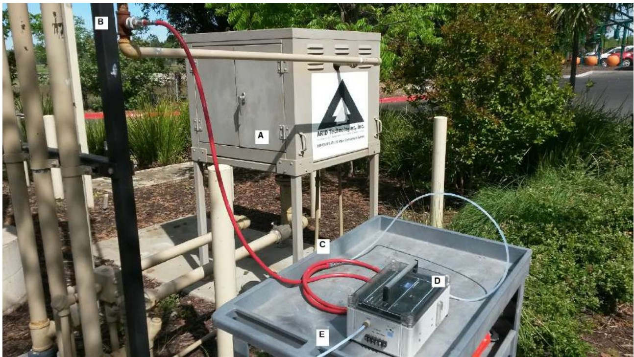
Figure 2 Equipment Configuration for Measuring Permeator Exhaust
