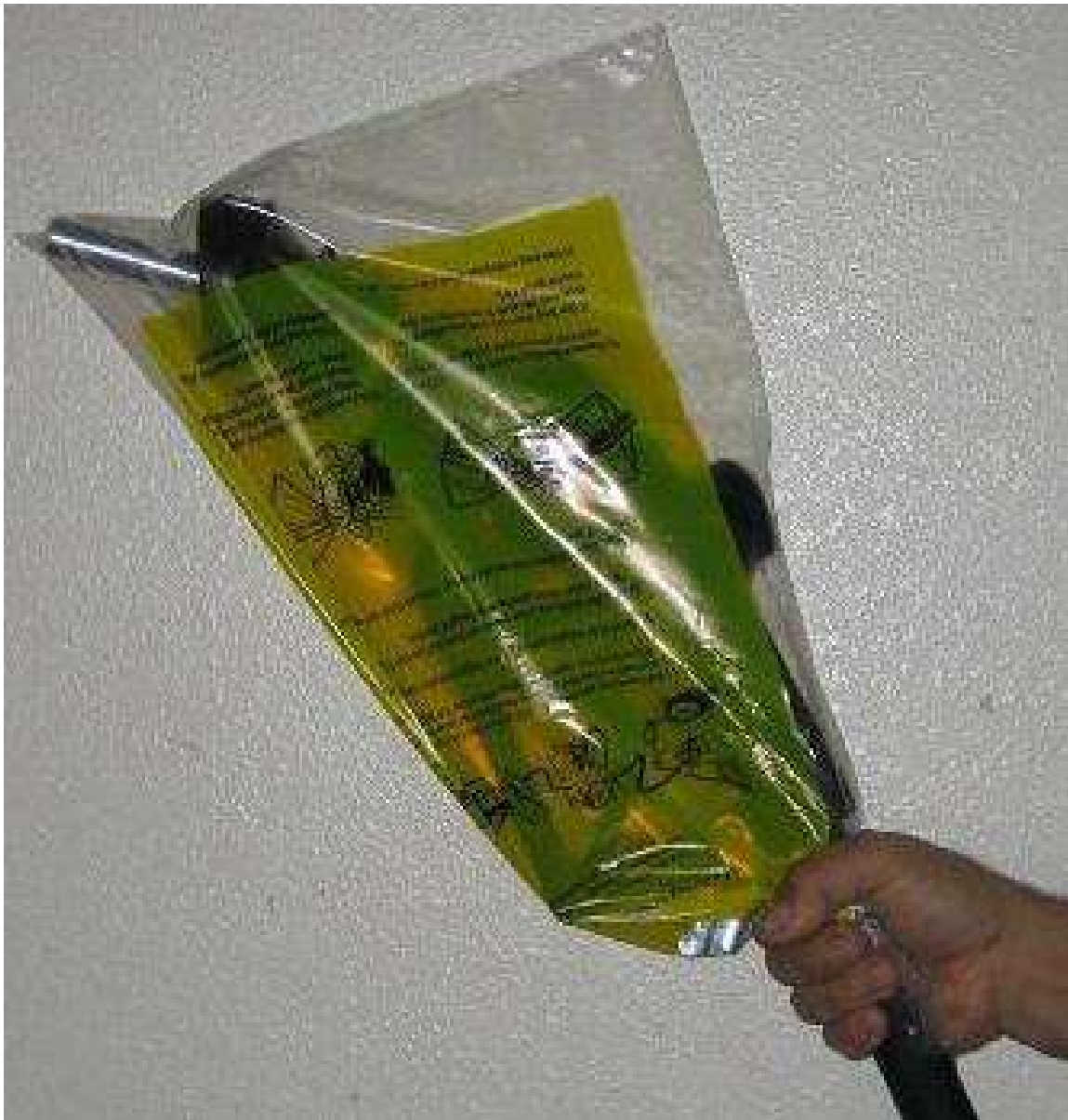
FIGURE 7-1 Typical Example of Bagging a Nozzle
