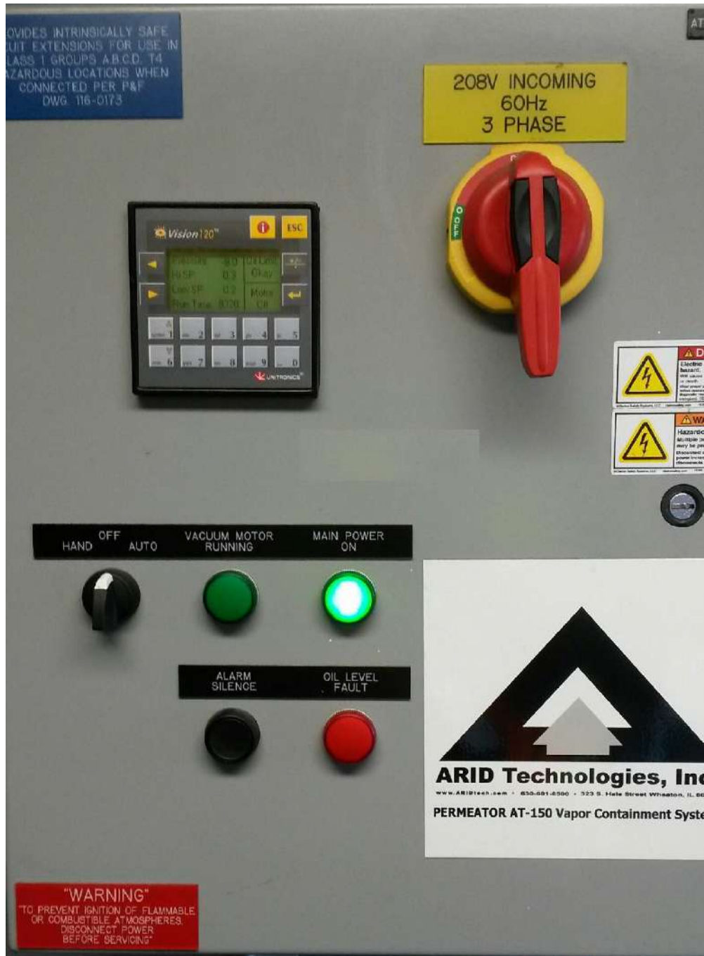
FIGURE 8-2 Configuration of Permeator Control Panel Hand/Off/Auto Control Knob in OFF position to Conduct TP-201.3
