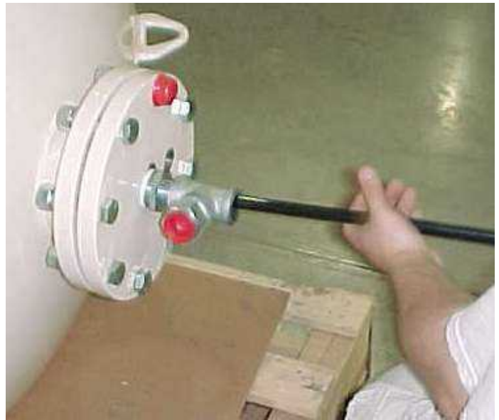
Figure 4: Install Syphon Tube
