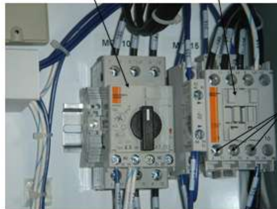
Motor Overload Breaker (6) and Motor Starter (7)
