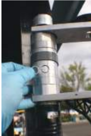
Figure 6: Add Shear Washer
