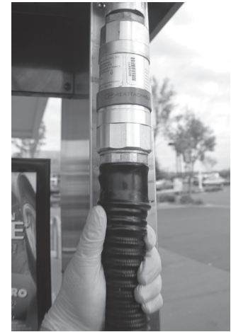
Figure 9: Verify Connection Integrity
