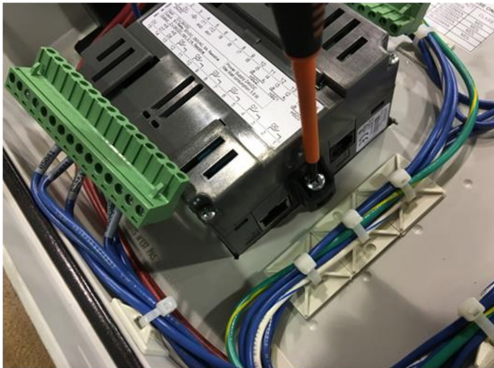
Removing the PLC Hold-Down Clips, 2-28-2018
