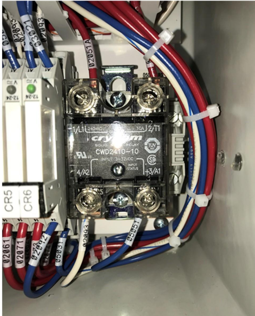
Figure 9-9: Vacuum Pump Solid State Relay
