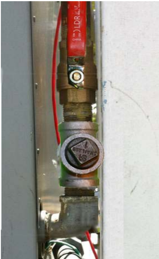
Figure 5: Ball Valve and 1" Plug on Test Port
