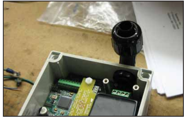
Figure 8: 90-Degree Fitting Installed
