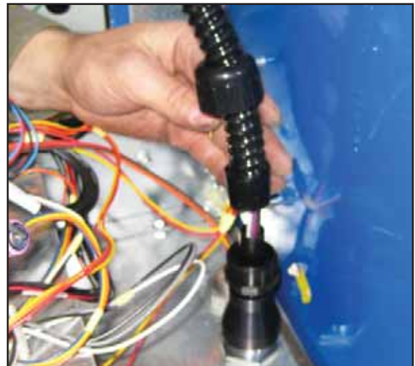
Figure 10: Wire in Flexible Conduit
