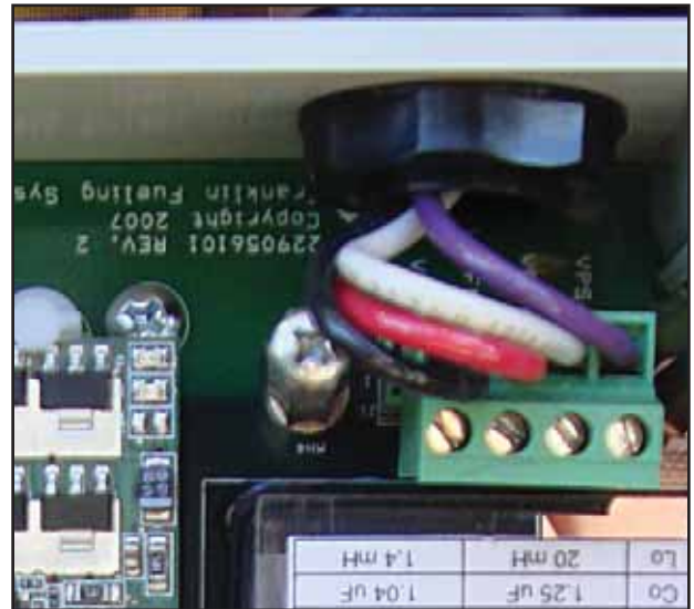
Figure 14: Wiring Connection to DTU
