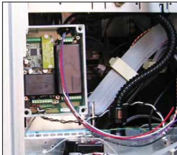
Figure 13: Wires in Flexible Conduit
