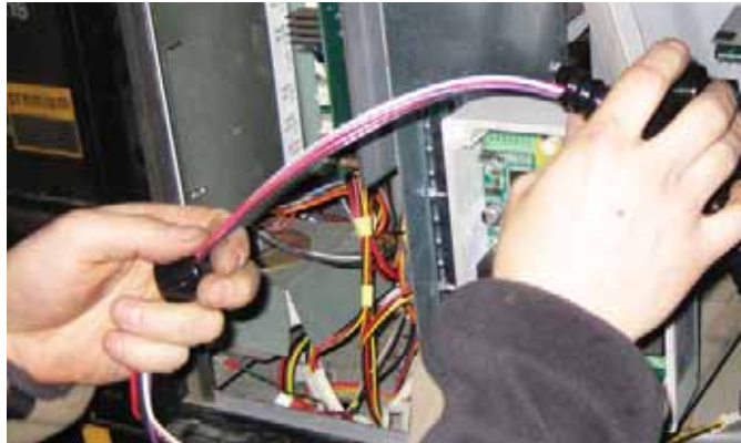
Figure 11: Attach Flexible Conduit to 90-Degree Fitting
