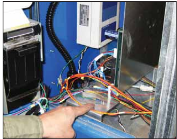
Figure 18: Ground Wire Attached
