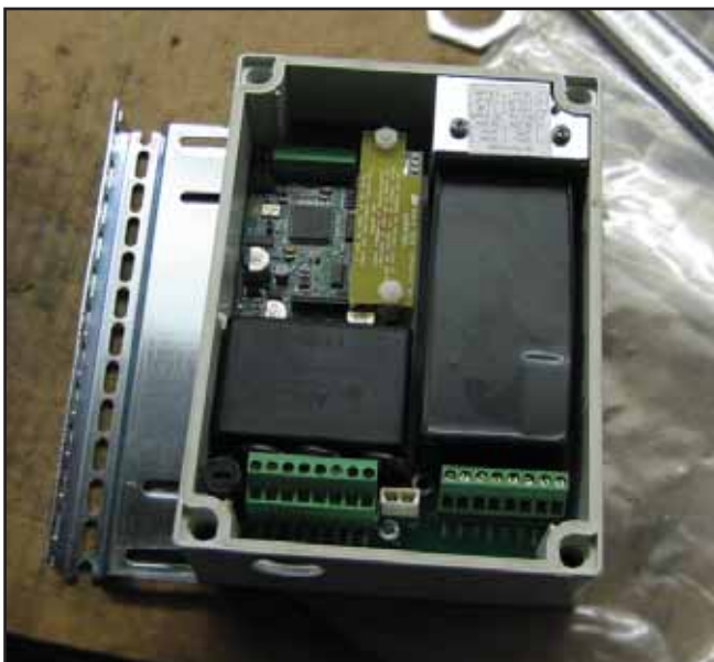
Figure 2: Mounting Bracket Installed
