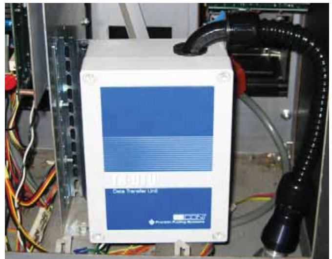
Figure 14: DTU Attached to Dispenser
