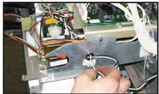
Figure 10: Power Harness Wiring
