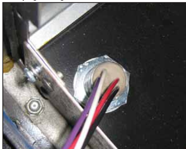
Figure 5: Potted Nipple Installed
