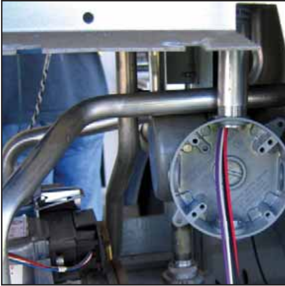
Figure 8: Junction Box Connected to Potted Nipple
