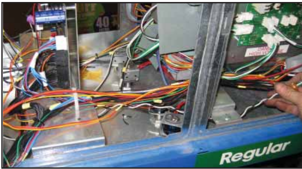
Figure 16: Power Cable Installation
