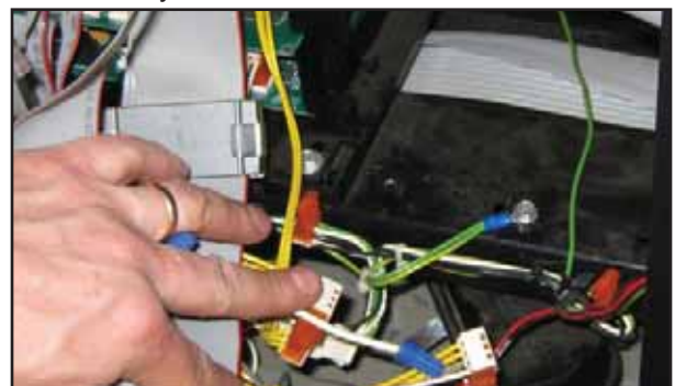
Figure 5: Reinstalled Ground Wire
