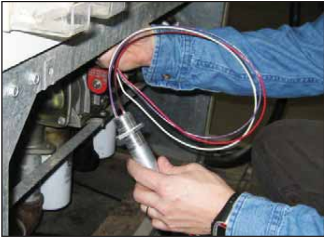
Figure 10: Push Wire to Electrical Enclosure
