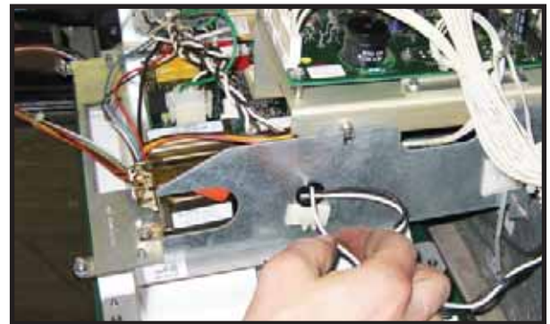
Figure 9: Power Harness Wiring
