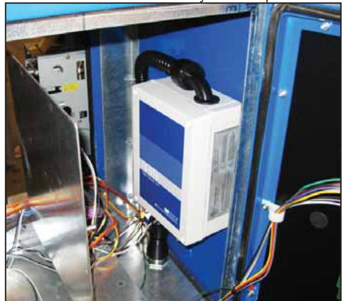
Figure 15: DTU Attached to Dispenser
