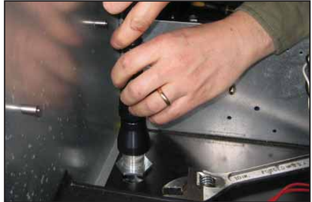
Figure 13: Attach Flexible Conduit
