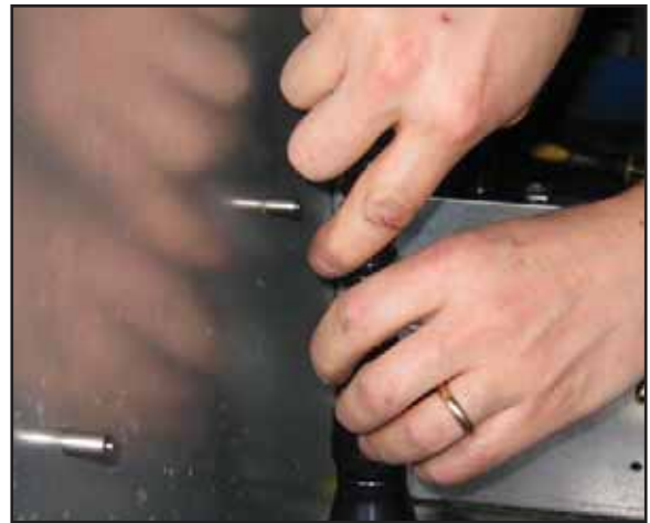
Figure 11: Flexible Conduit Installation
