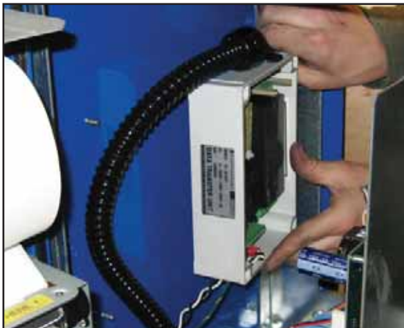
Figure 13: 90-Degree Conduit Connected
