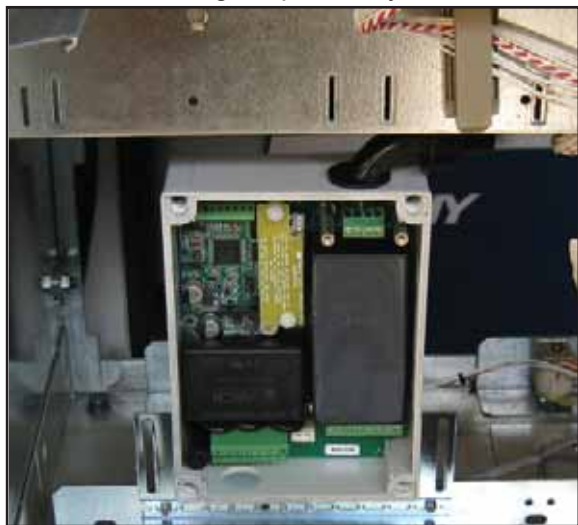
Figure 11: 90-degree Fitting Installed
