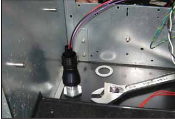
Figure 6: Straight Conduit Installed
