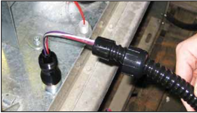
Figure 14: Attach Flexible Conduit to Potted Nipple
