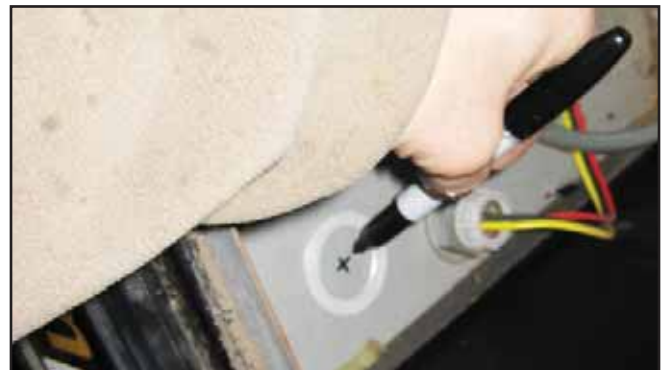
Figure 5: Mark Drilling Location
