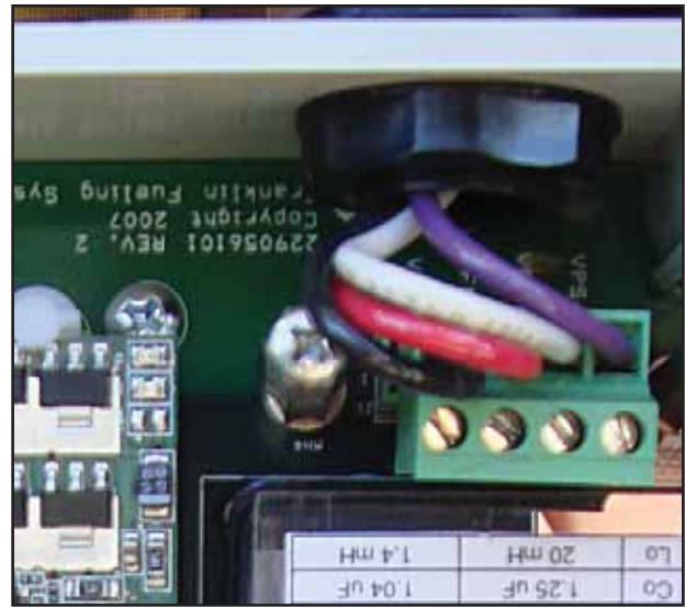
Figure 12: Wiring Connection to DTU
