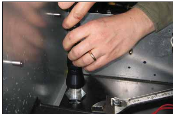
Figure 14: Attach Flexible Conduit
