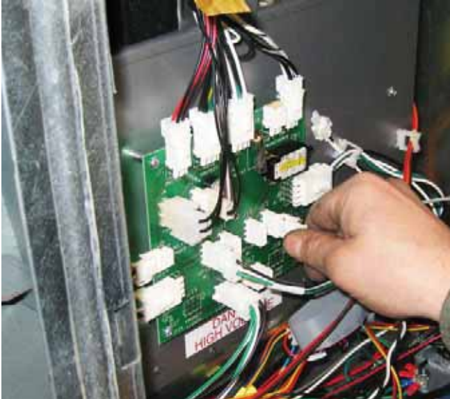
Figure 15: Connect to AC Power Board
