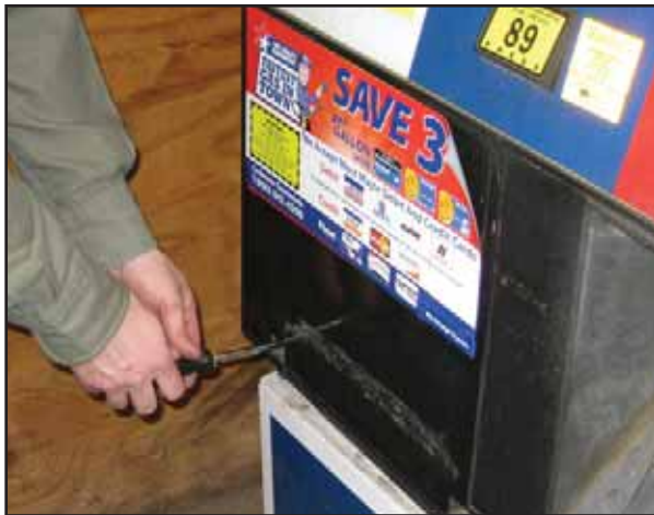
Figure 1: Loosen Bolts
