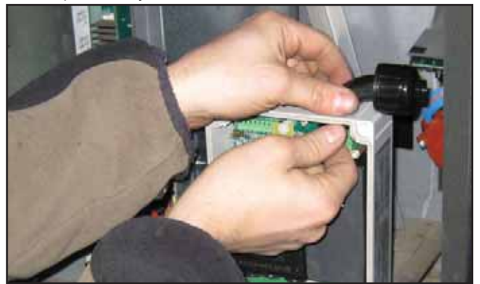
Figure 9: Attach 90-degree Fitting
