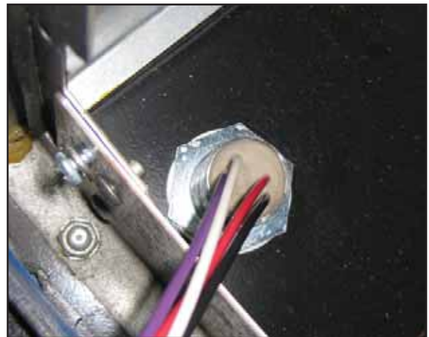
Figure 4: Potted Nipple Installed
