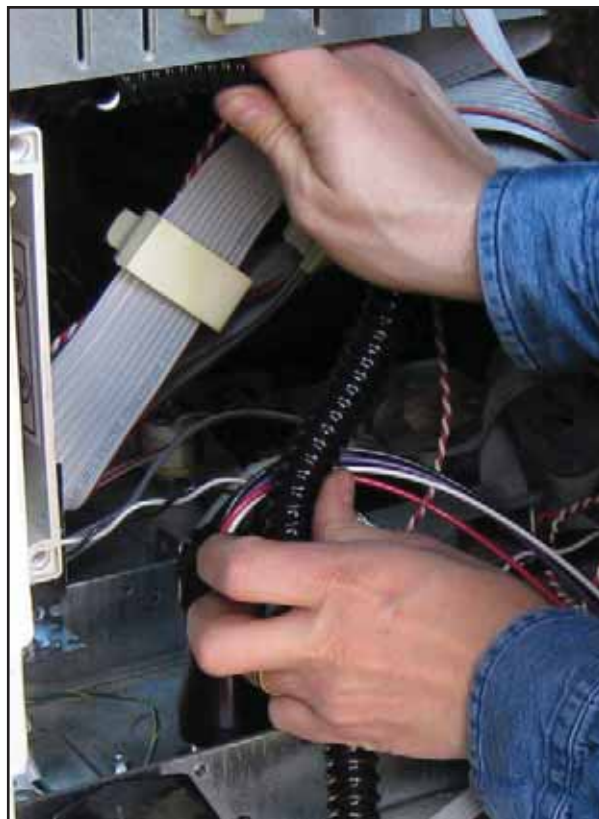
Figure 12: Flexible Conduit Installation
