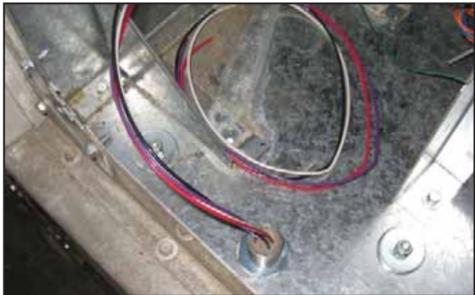
Figure 11: Install Potted Nipple
