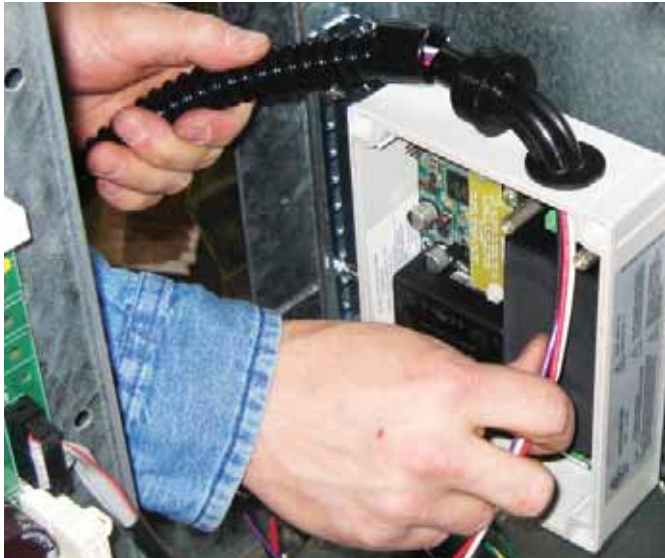
Figure 15: Attach Flexible Conduit to 90-Degree Fitting
