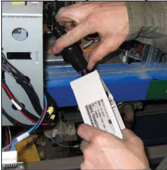
Figure 12: Pull wires through 90-degree fitting
