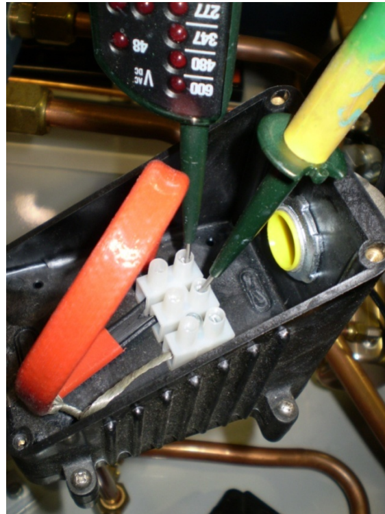
Figure 16: Heat Trace Circuit Test
