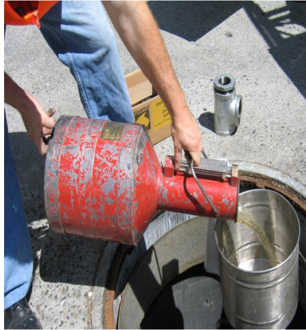
FIGURE 11-3 Adding Gasoline through Open Fuel Entry Point
