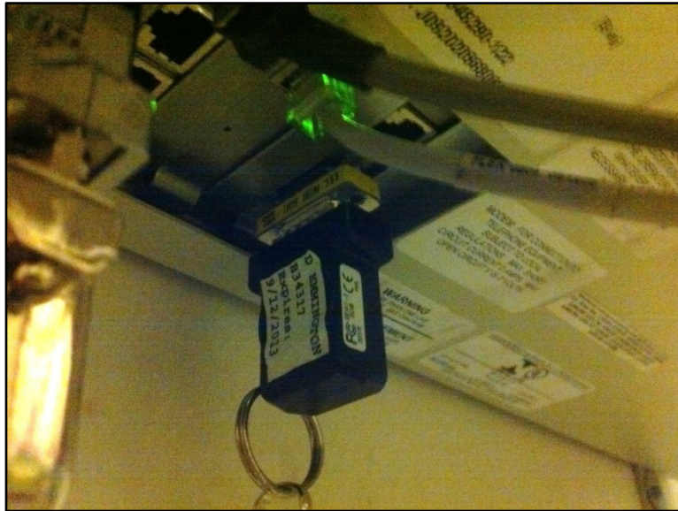
FIGURE 4 Maintenance Tracker Key Plugged Into TLS Console
