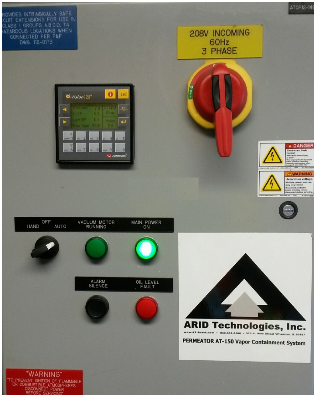
FIGURE 8-3 Configuration of Permeator Control Panel Hand/Off/Auto Control Knob in AUTO position after Conducting TP-201.3
