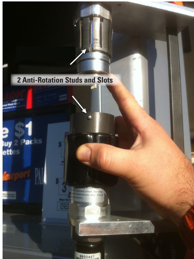
Figure 3. Anti-Rotation Studs and Slots
