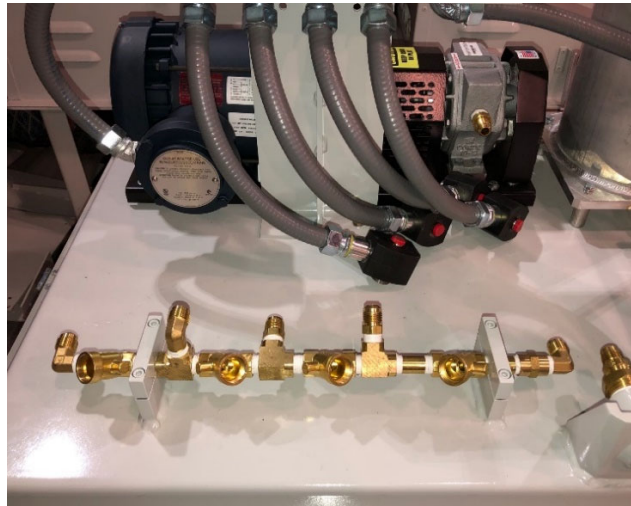
Figure 9-29: Solenoids (with the Solenoid Bases Installed) Arranged Out of the Way
