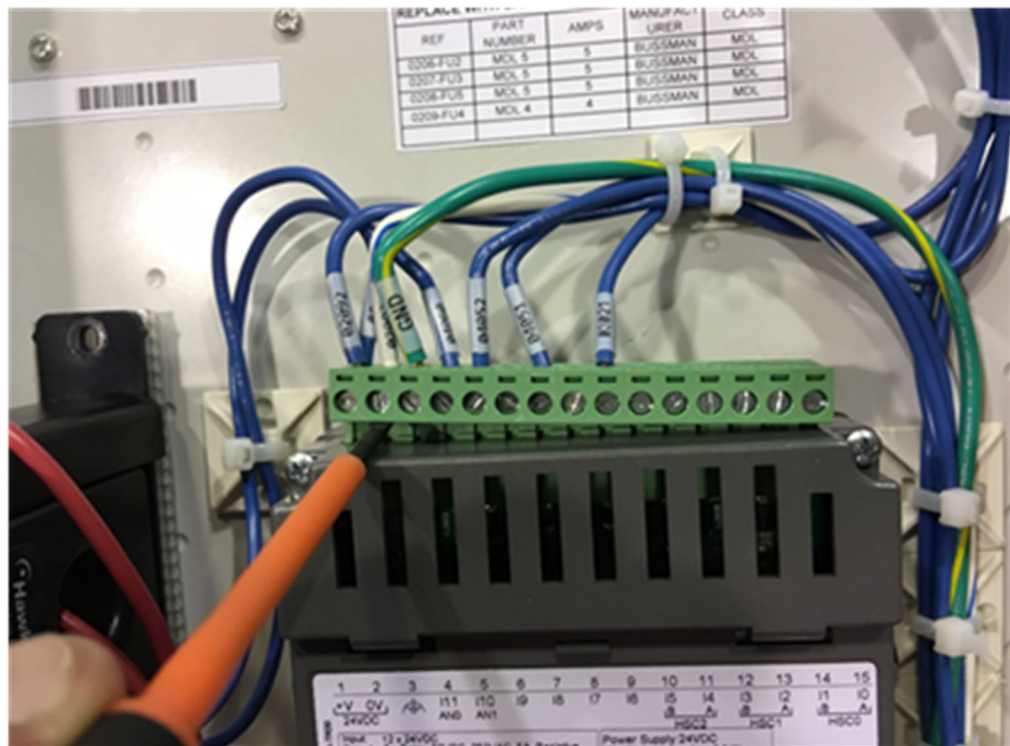
Removing the PLC Connectors, 2-28-2018
