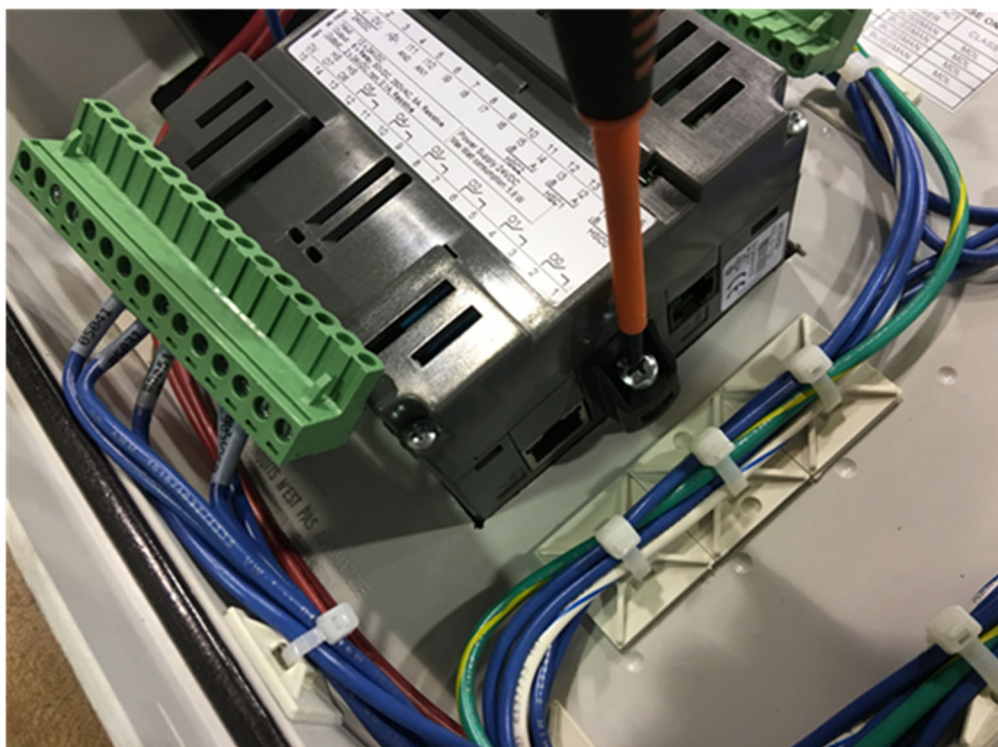
Removing the PLC Hold Down Clips, 2-28-2018
