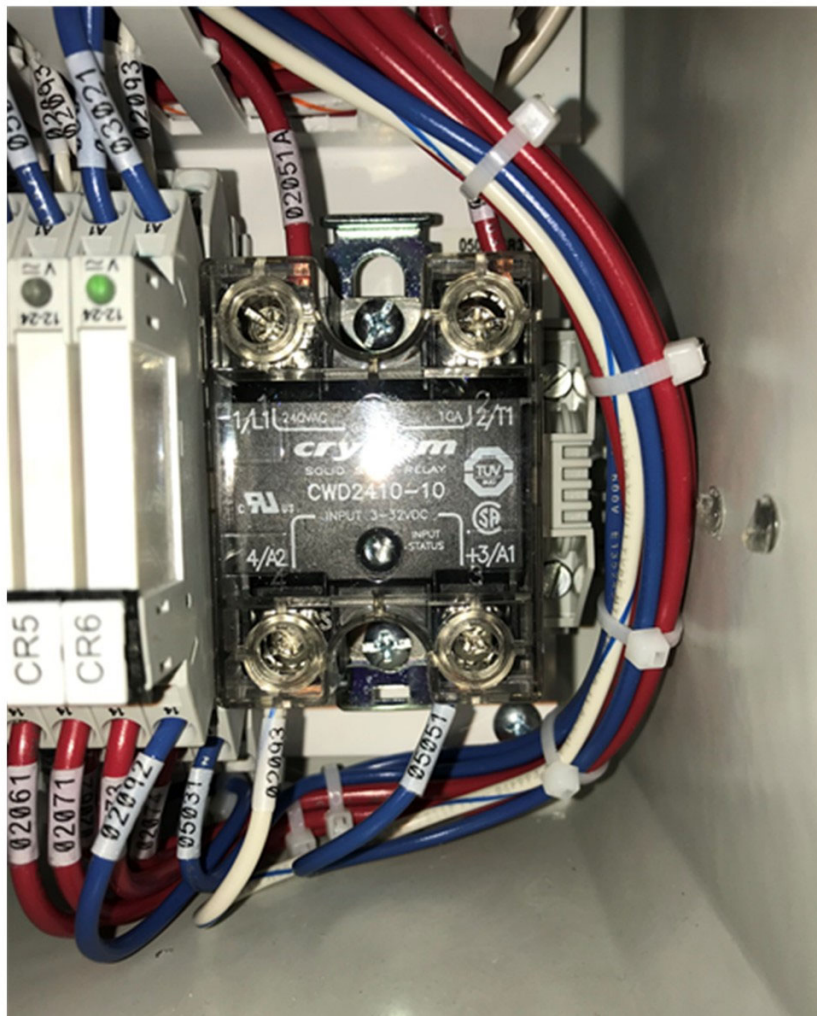
Figure 9-9: Vacuum Pump Solid State Relay
