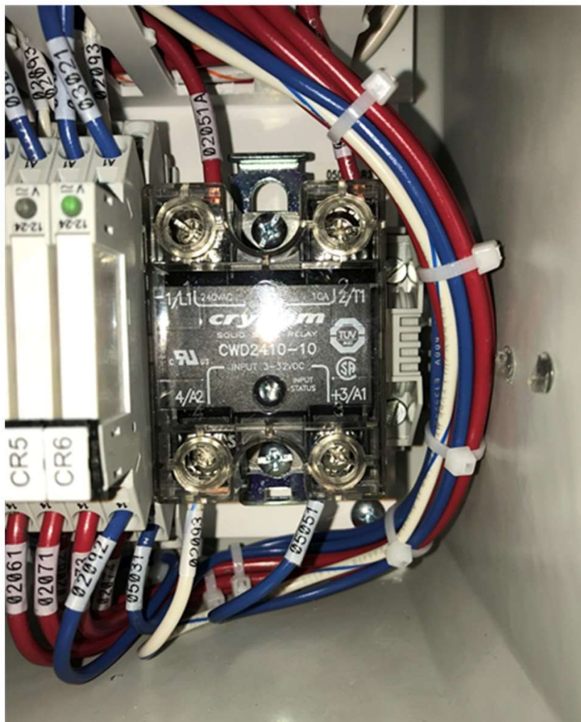
Figure 9-9: Vacuum Pump Solid State Relay
