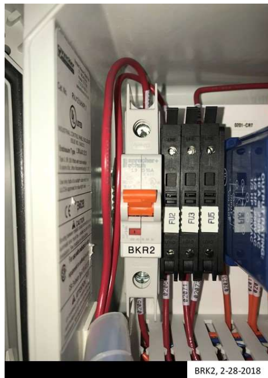
Figure 9-8: Vacuum Pump BRK2
