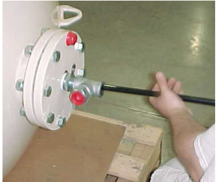
Figure 4: Install Syphon Tube
