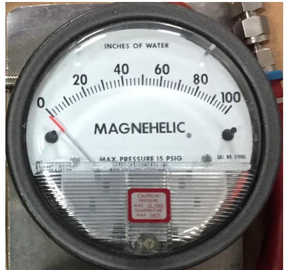
Typical Mechanical Gauges
