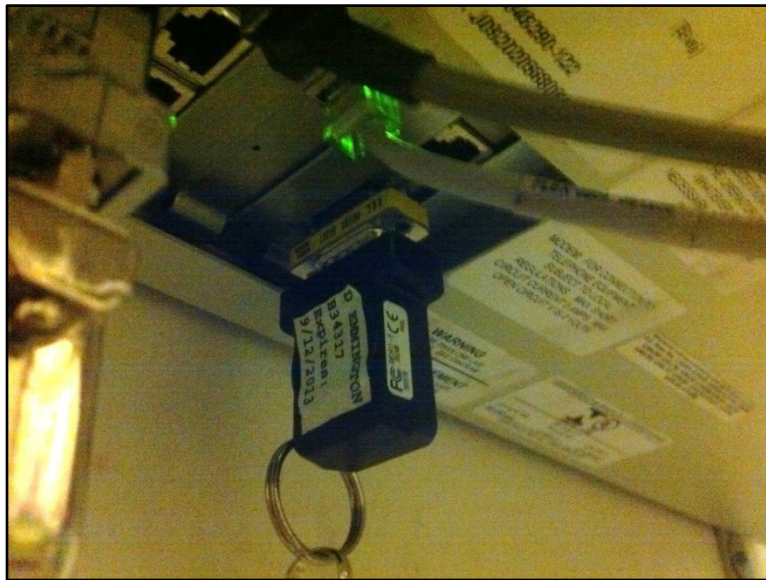
FIGURE 4 Maintenance Tracker Key Plugged Into TLS Console
