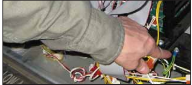
Figure 4: Find Ground Wire
