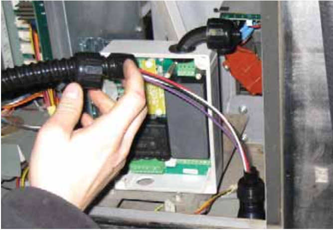
Figure 10: Attach Flexible Conduit to Potted Nipple
