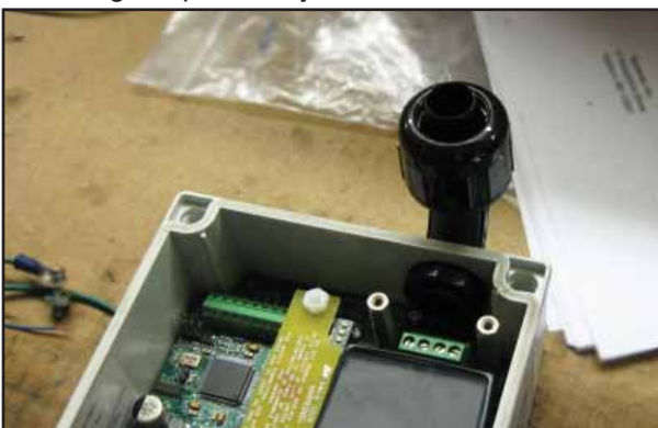
Figure 7: 90-Degree Fitting Installed
