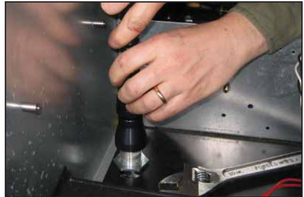
Figure 13: Attach Flexible Conduit
