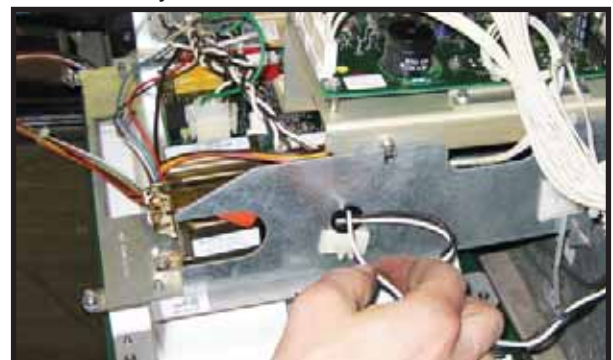
Figure 10: Power Harness Wiring
