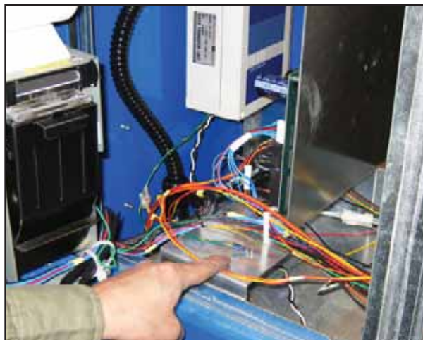
Figure 18: Ground Wire Attached
