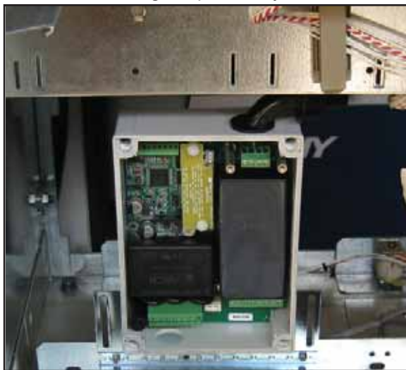
Figure 11: 90-degree Fitting Installed
