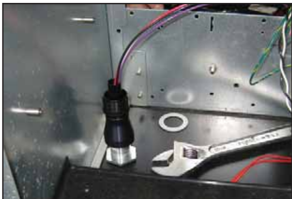
Figure 5: Straight Conduit Installed
