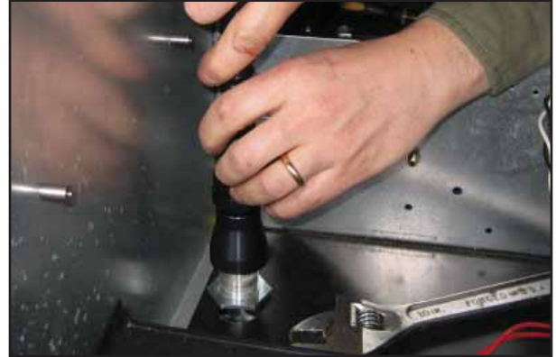
Figure 14: Attach Flexible Conduit
