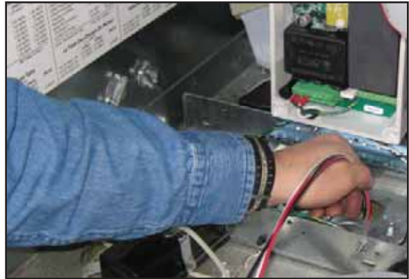
Figure 8: Pulling Wires Through Opening
