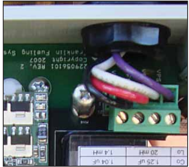
Figure 12: Wiring Connection to DTU
