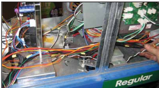
Figure 16: Power Cable Installation
