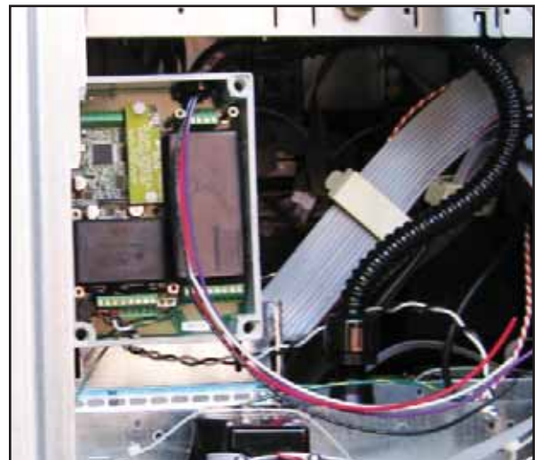
Figure 13: Wires in Flexible Conduit
