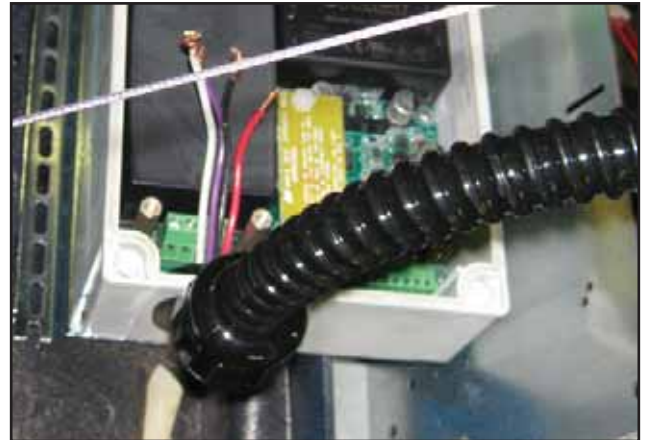
Figure 12: 90-Degree Fitting Installed
