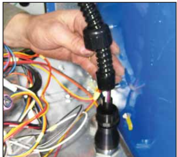
Figure 10: Wire in Flexible Conduit
