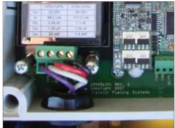
Figure 13: Wires attached to DTU
