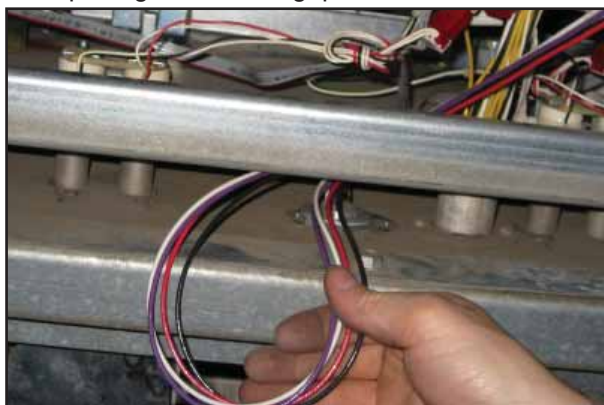
Figure 8: Potted Conduit wires
