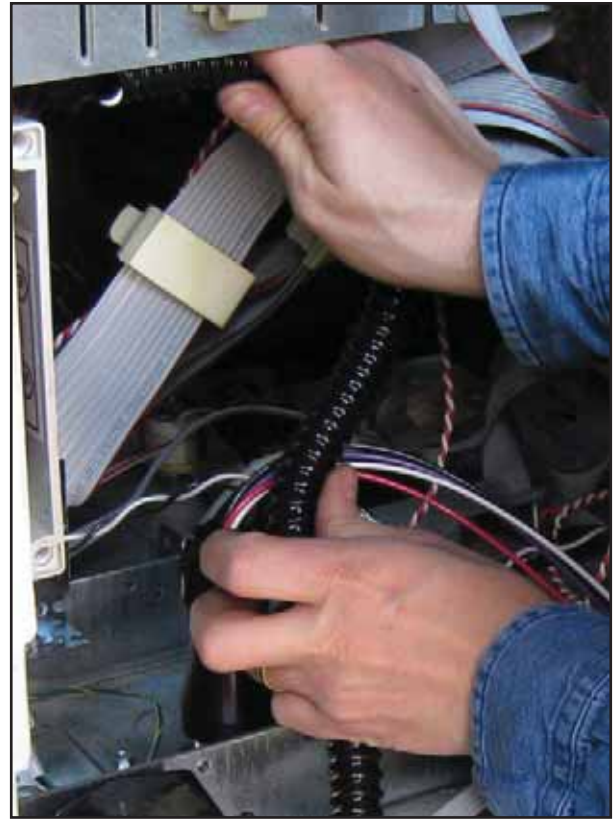
Figure 12: Flexible Conduit Installation
