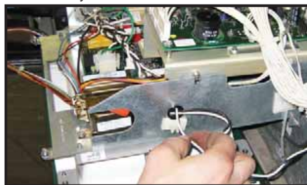
Figure 9: Power Harness Wiring
