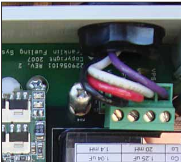
Figure 14: Wiring Connection to DTU
