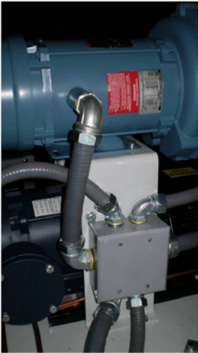
Figure 23: Blower electrical connection conduit
