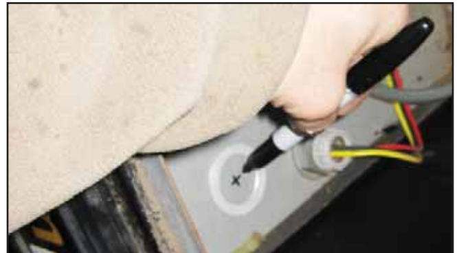
Figure 5: Mark Drilling Location
