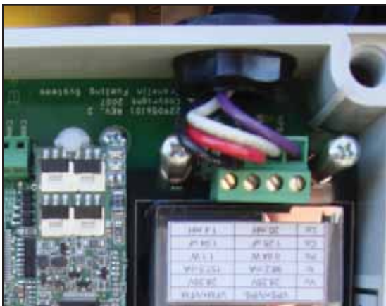
Figure 16: Terminal Block Wiring
