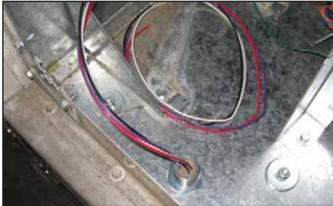
Figure 11: Install Potted Nipple
