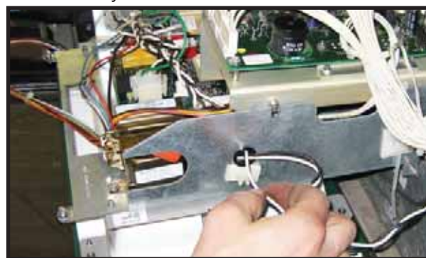
Figure 9: Power Harness Wiring
