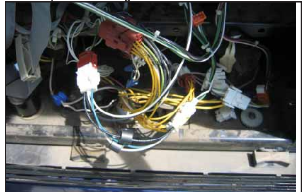
Figure 4: Power Distribution Wires
