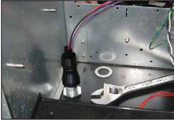
Figure 6: Straight Conduit Installed
