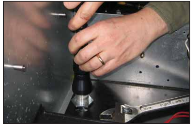
Figure 13: Attach Flexible Conduit
