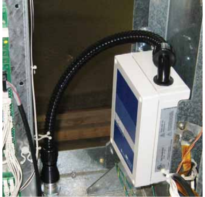
Figure 17: Attach Cover to DTU
