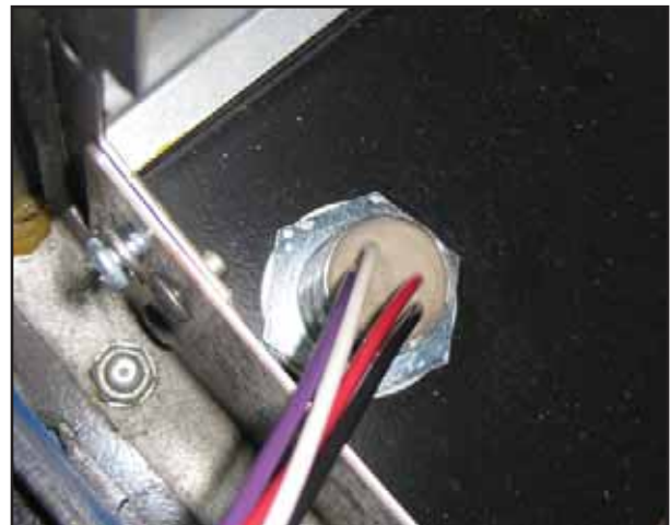
Figure 5: Potted Nipple Installed
