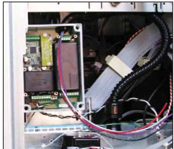
Figure 13: Wires in Flexible Conduit
