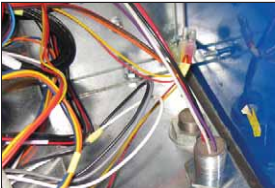
Figure 8: Potted Nipple Installed
