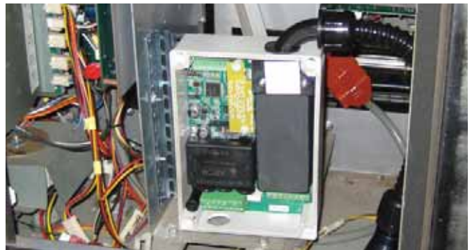
Figure 13: Reinstall Barrier Cover
