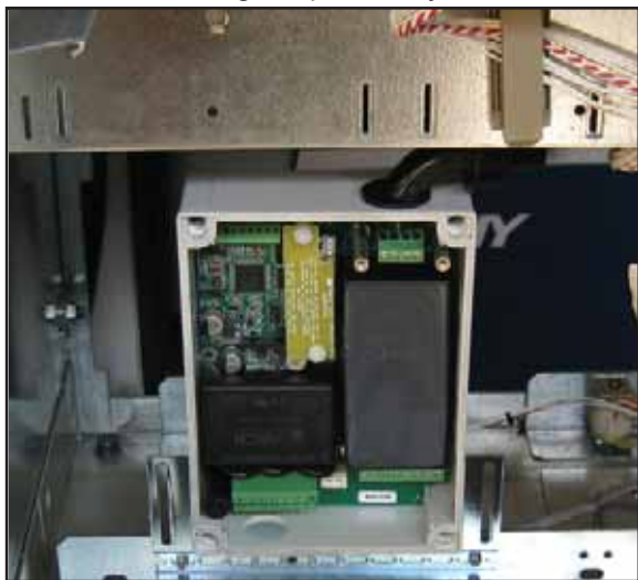
Figure 11: 90-degree Fitting Installed
