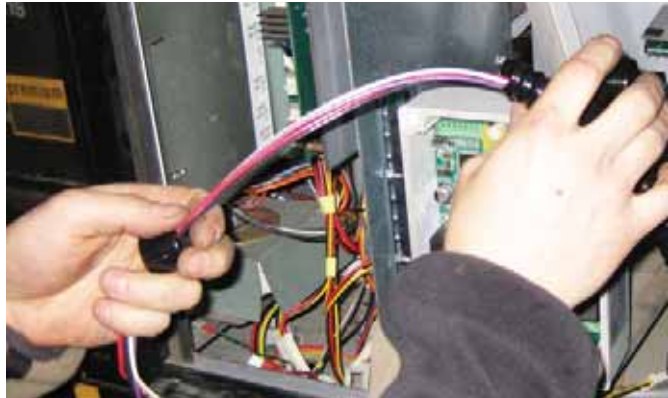
Figure 11: Attach Flexible Conduit to 90-Degree Fitting
