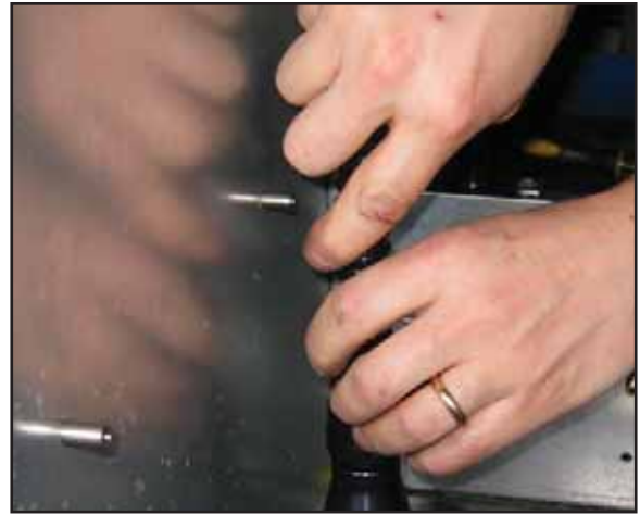
Figure 11: Flexible Conduit Installation
