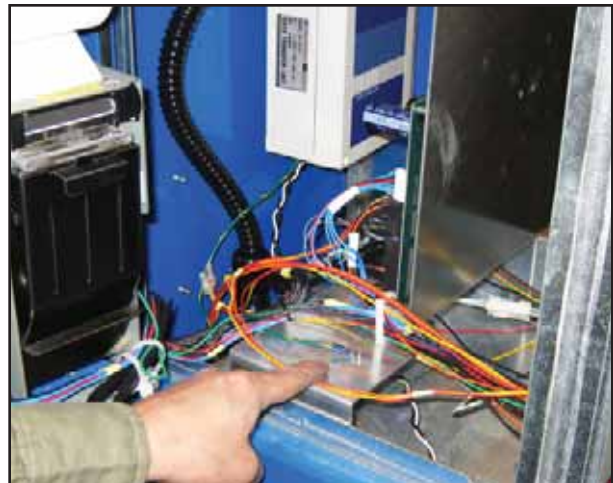
Figure 18: Ground Wire Attached
