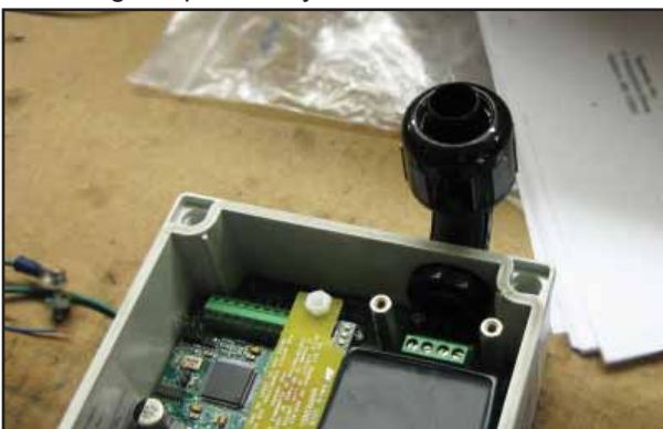
Figure 7: 90-Degree Fitting Installed
