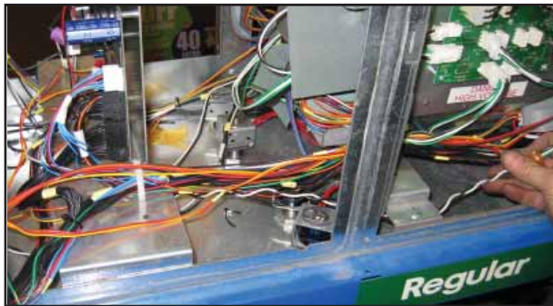
Figure 16: Power Cable Installation
