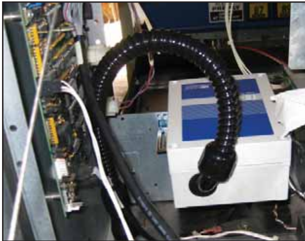
Figure 17: DTU Installed with Cover On
