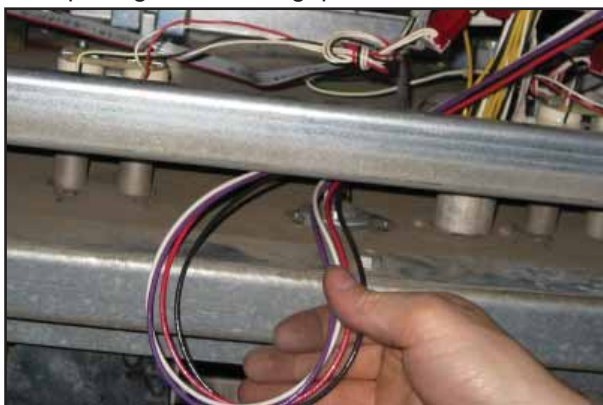
Figure 8: Potted Conduit wires
