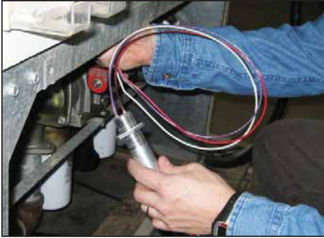
Figure 10: Push Wire to Electrical Enclosure
