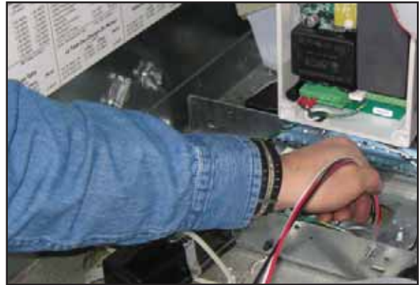
Figure 8: Pulling Wires Through Opening
