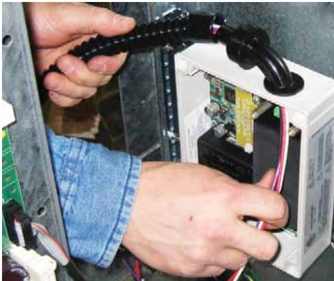
Figure 15: Attach Flexible Conduit to 90-Degree Fitting
