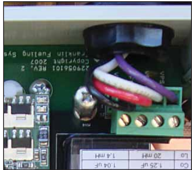
Figure 12: Wiring Connection to DTU
