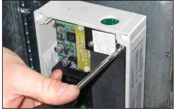
Figure 12: Remove Wiring Cover
